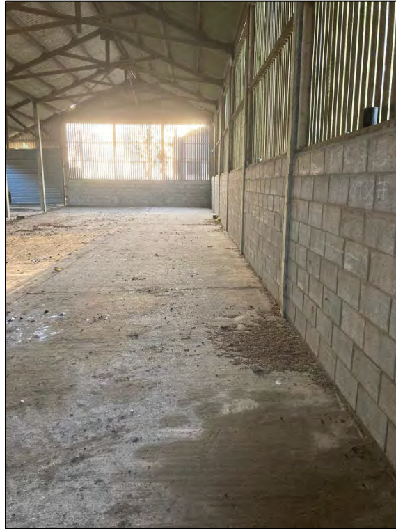
Photograph 5: Inside the barn, looking towards the front (and west).
