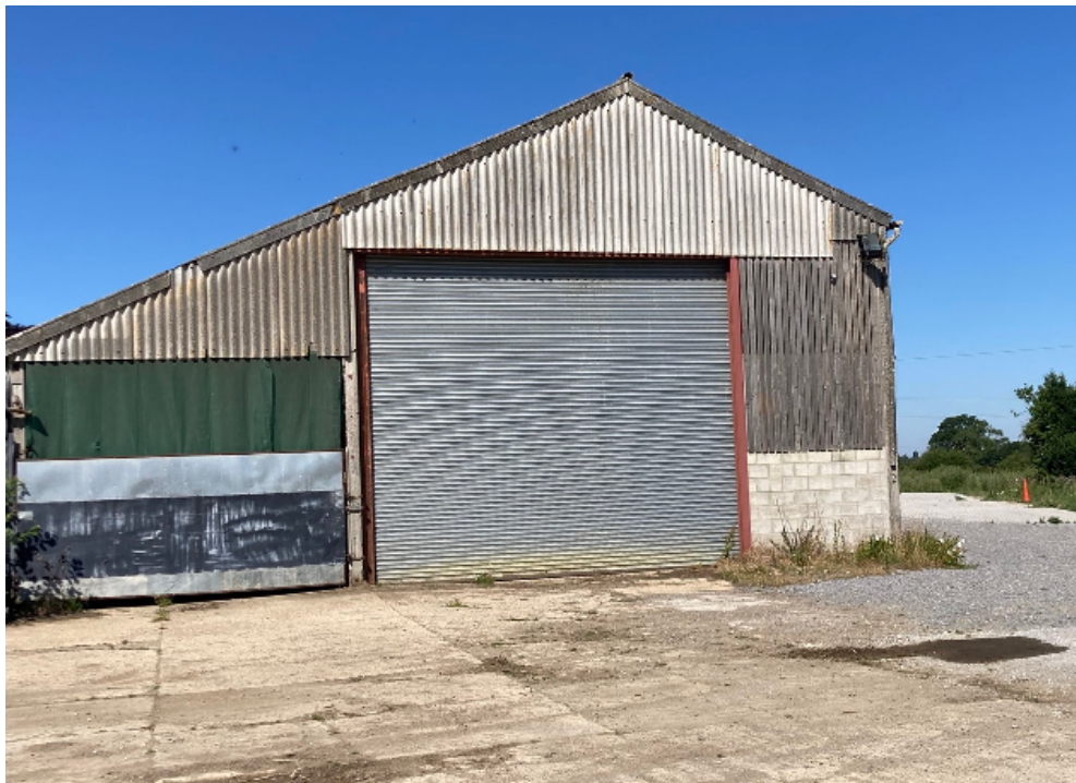
Photograph 10: The rear / eastern side of the barn.
