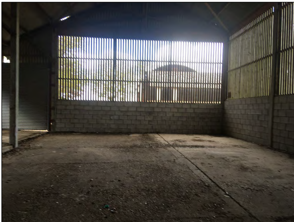
Photograph 6: Inside the barn, looking towards the front (and west).
