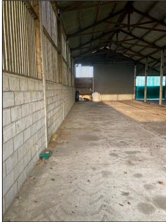
Photograph 7: Inside the barn, looking towards the rear (and east).
