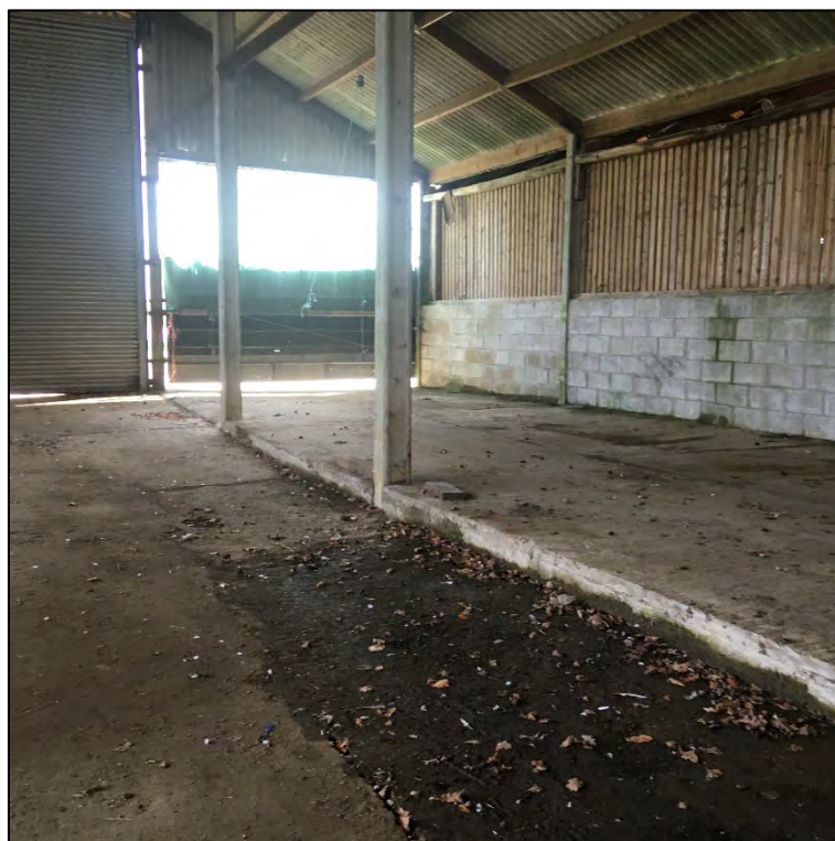
Photograph 8: Inside the barn, looking towards the rear (and east).
