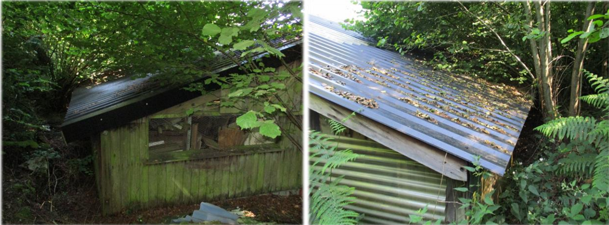
Storage barn rear elevation looking south (left) and looking north (right)
