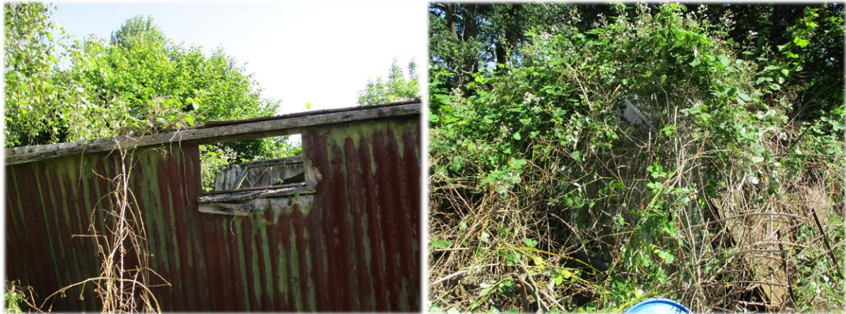
Dilapidated waggon with no roof (left) and a small greenhouse covered in bramble (right)
