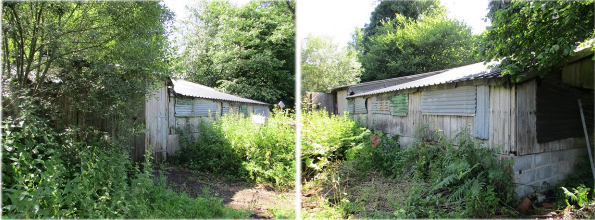
Storage barn front elevation looking south (left) and looking north (right)
