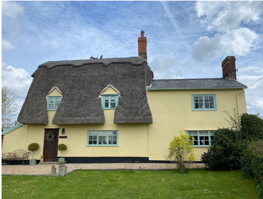
The original thatch inn with C19 slate addition.
