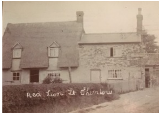
The unrendered C19 addition can be seen with a doorway to a possible second dwelling
