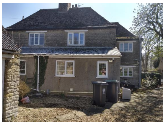
View of existing rear extension
