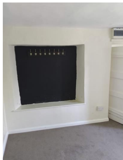
View of existing infilled opening ⑤
