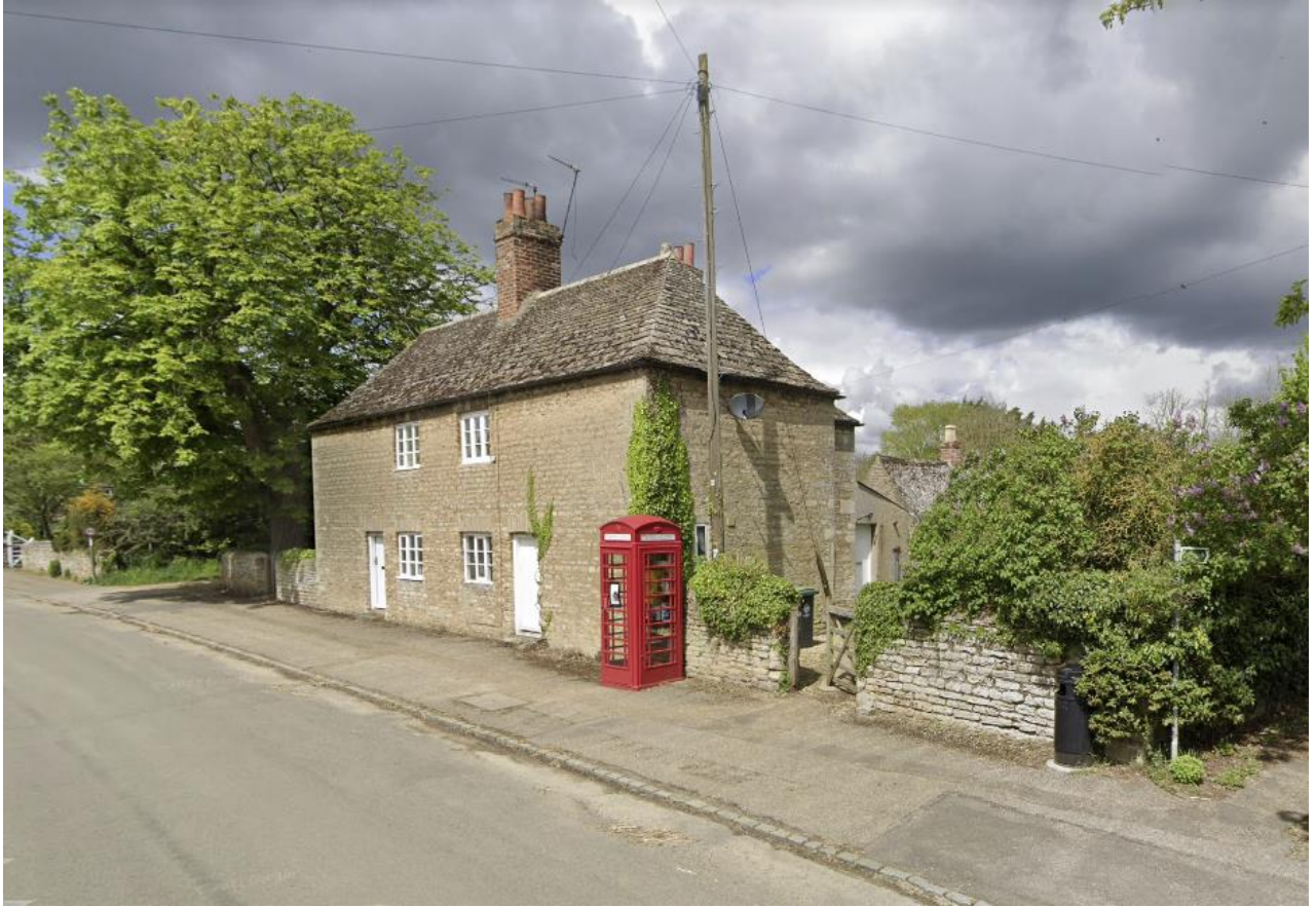
View looking west towards Nos. 26 & 27 Main Street
