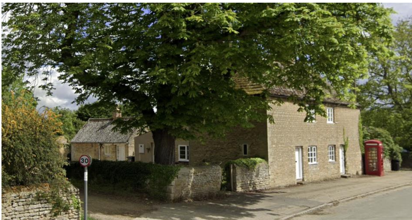
View looking east towards Nos. 26 & 27 Main Street
