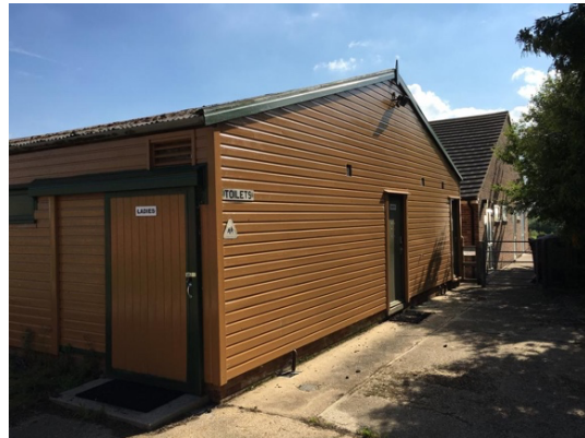
Existing Building toilet doors.
