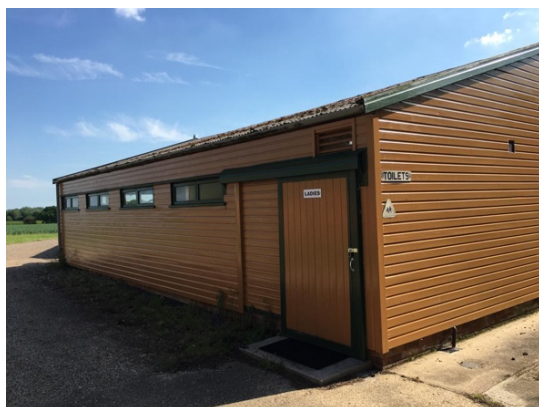
Existing Building exterior.
