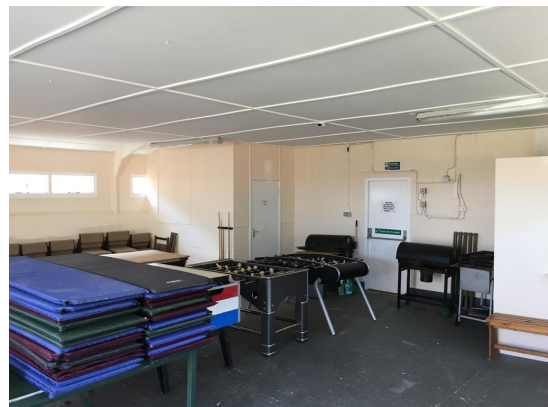
Existing Building Interior.
