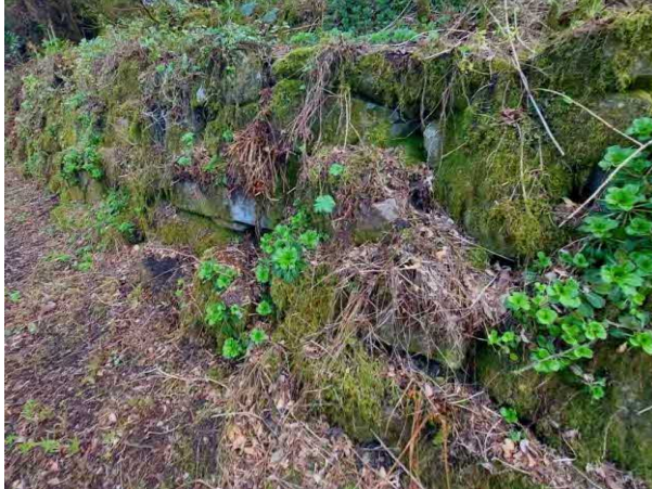
Photo 33: Stone wall gap
