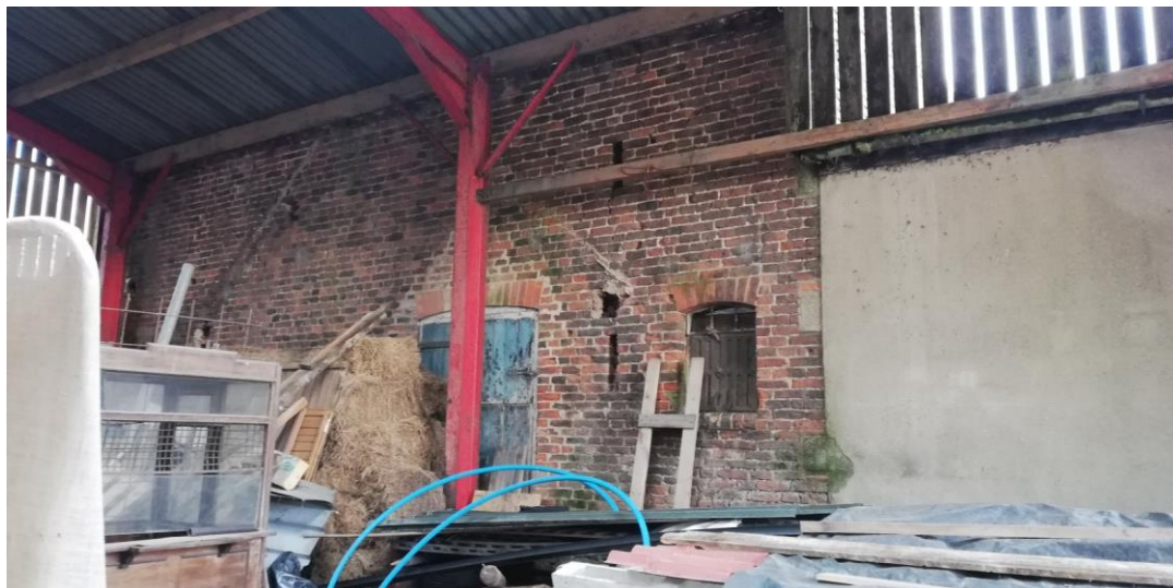
West Elevation viewed from within adjacent Barn
