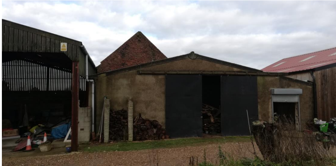
Exterior View from South
