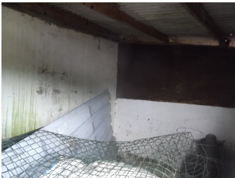
Plate 9. The interior of one of the pens of Building 3.
