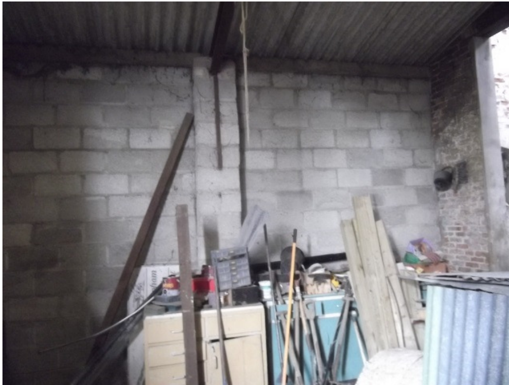
Plates 3 & 4. Internal views of Building 1.
