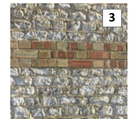
Existing External Barn Walls And Materials Retained As Existing
