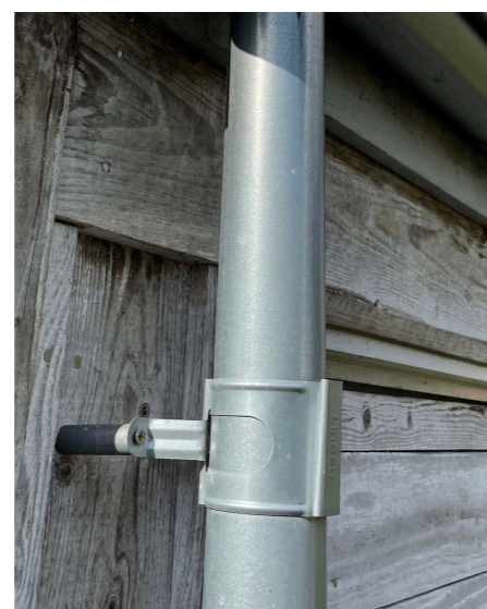
Galvanised metal downpipes
