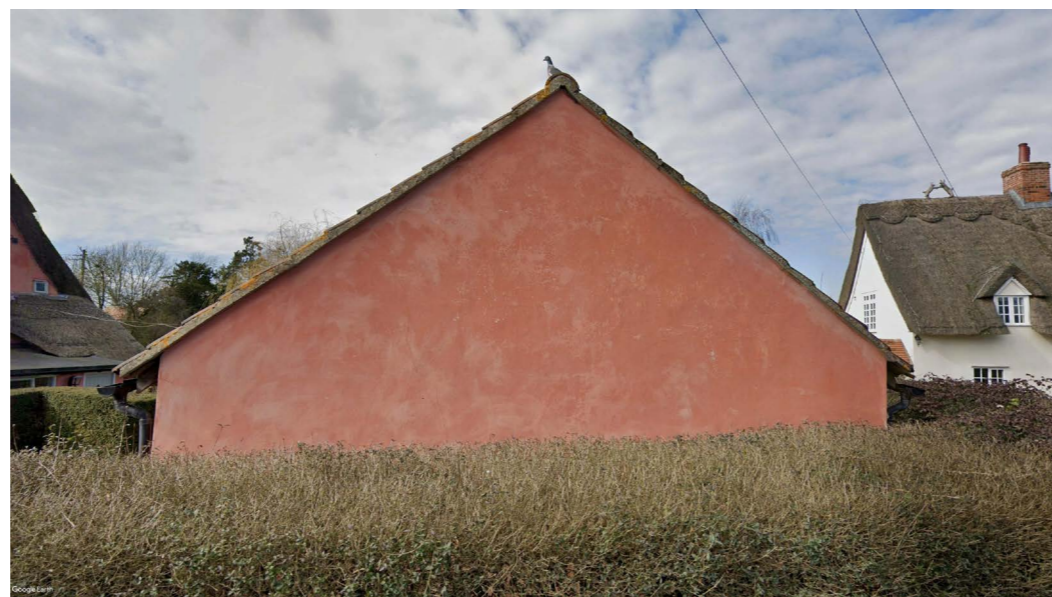
View from streetside showing East Elevation
