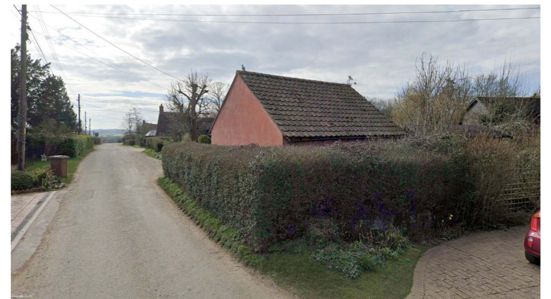
View from streetside approaching from Rear
