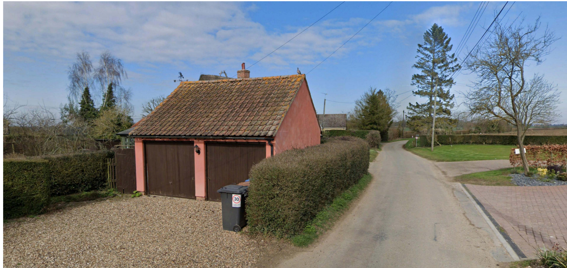
View from street approaching the garage doors
