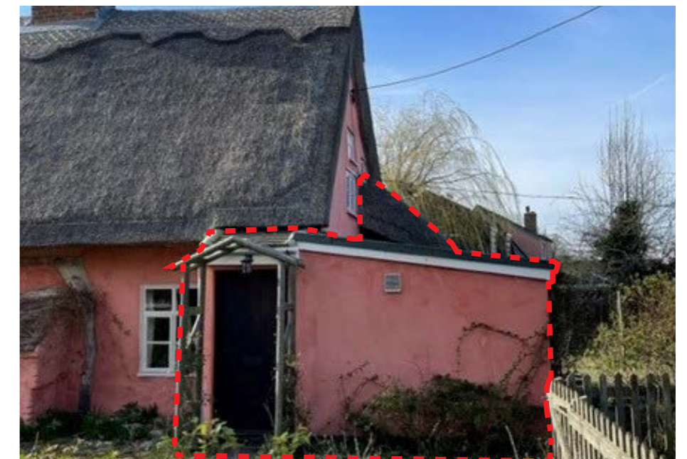
View3- Porch to be demolished..
