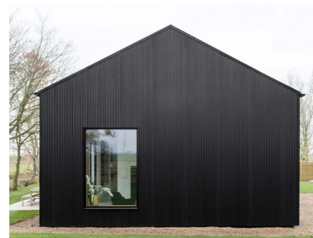
Examples of Black Stained Timber Barns in Suffolk Area
