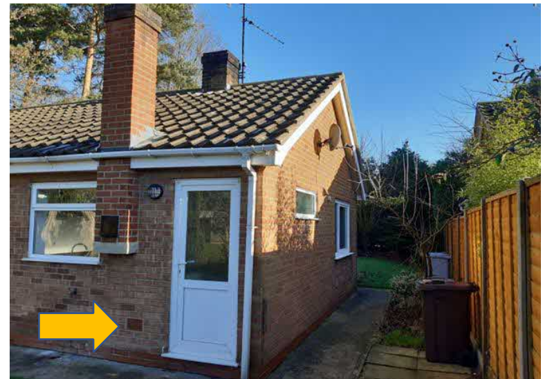
View of lower vent in rear elevation.
