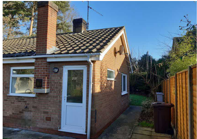
View of rear [redacted] and south boundary looking east..
