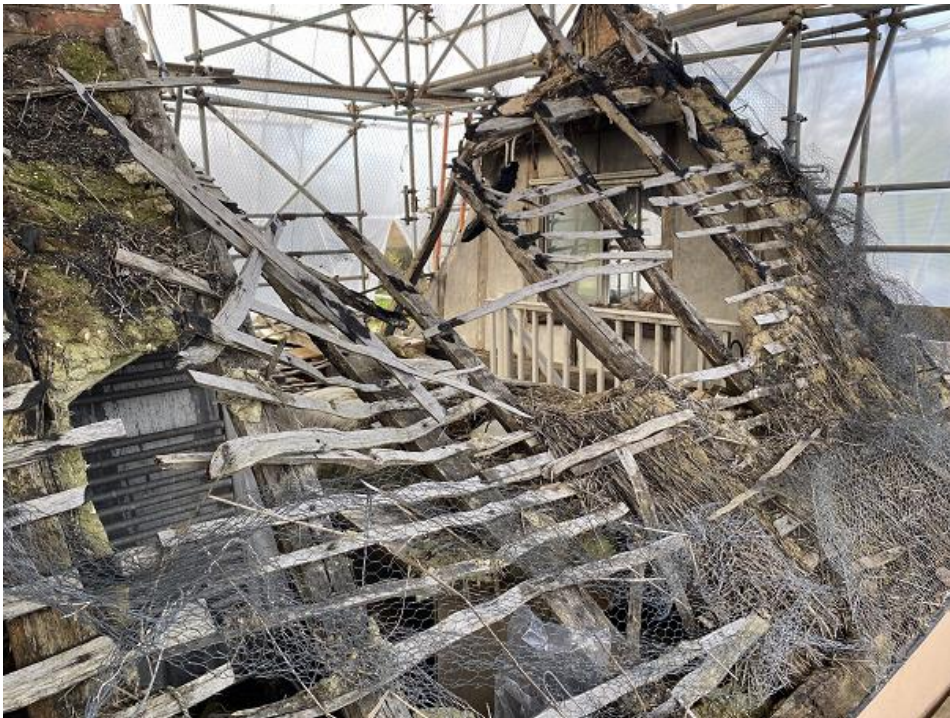
Figure 9: View of roof structure over the C18 range
