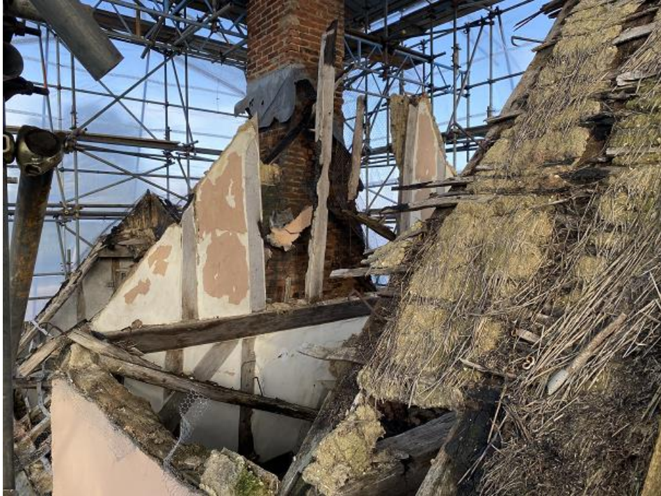
Figure 8: View looking north showing north gable frame of C16 range
