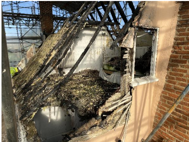
Figure 8: View of attic in C16 range
