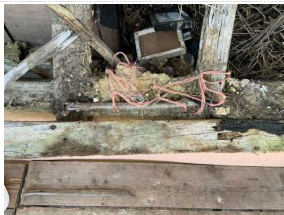
Plate 4. Branches used as battens.
