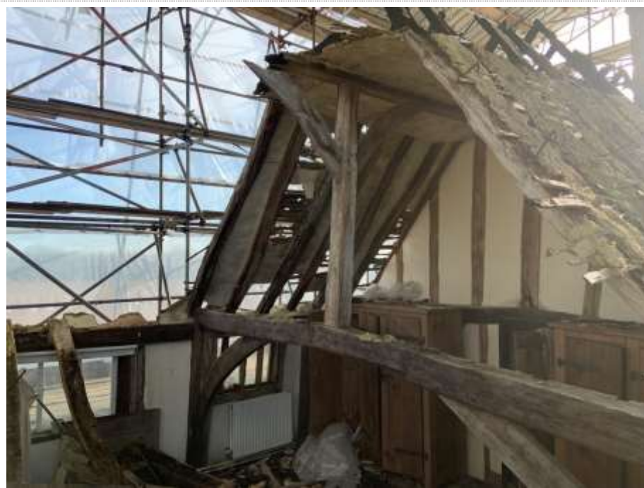
Plate 9. Roof 2 – Middle roof with 2-dimensional frame.
