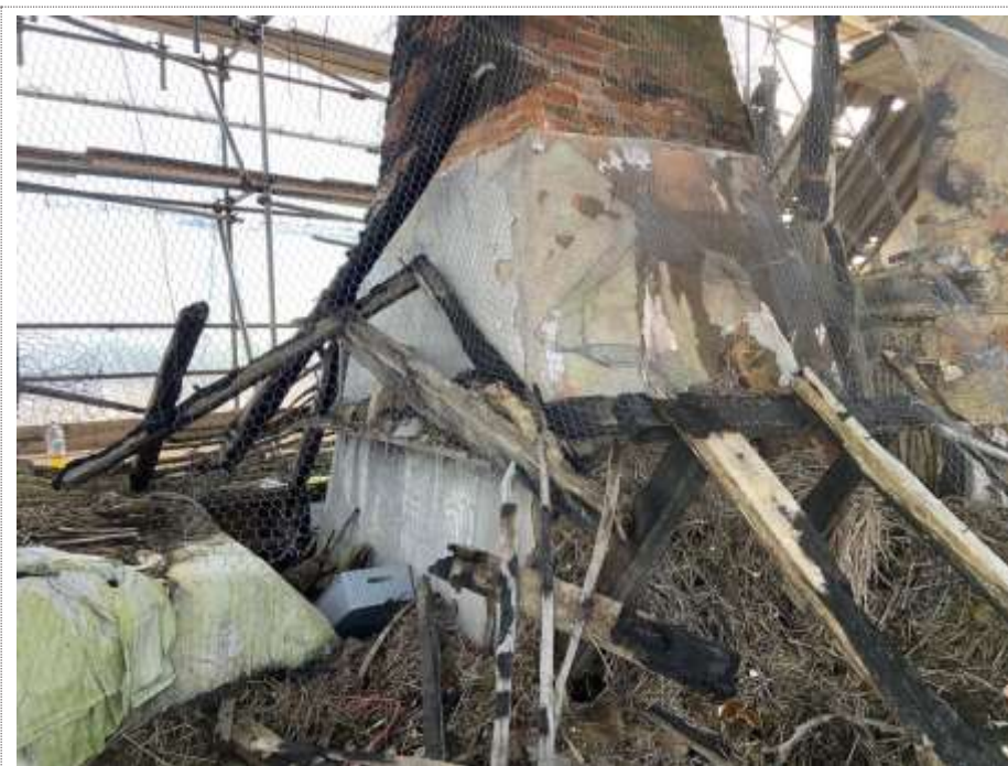
Plate 5. Bracing around the chimney structure.
