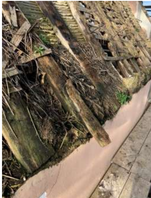
Plate 18. More modern lath and plaster finish on Roof 3 compared to Roof 2.
