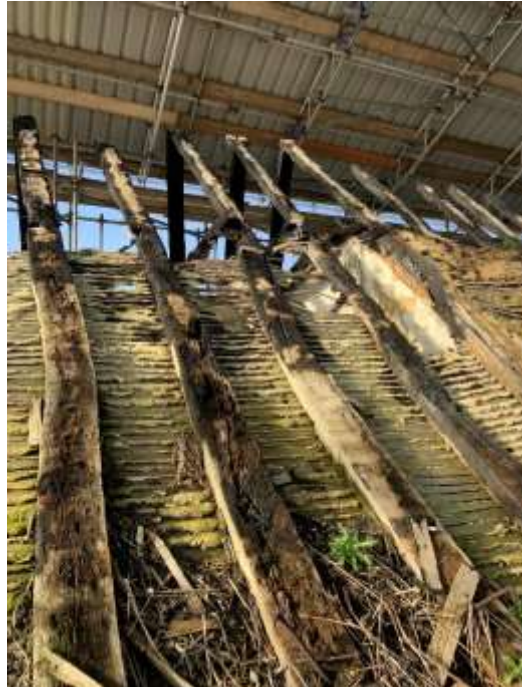
Plate 17. Vegetation growing at the back of Roof 3.
