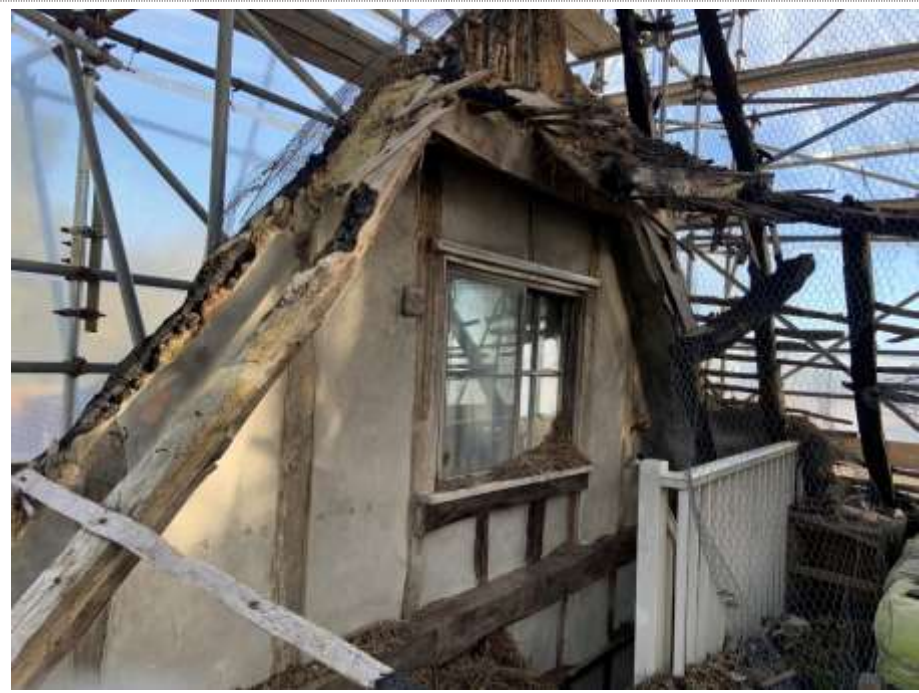
Plate 3. Roof 1 – Lower left-hand side.
