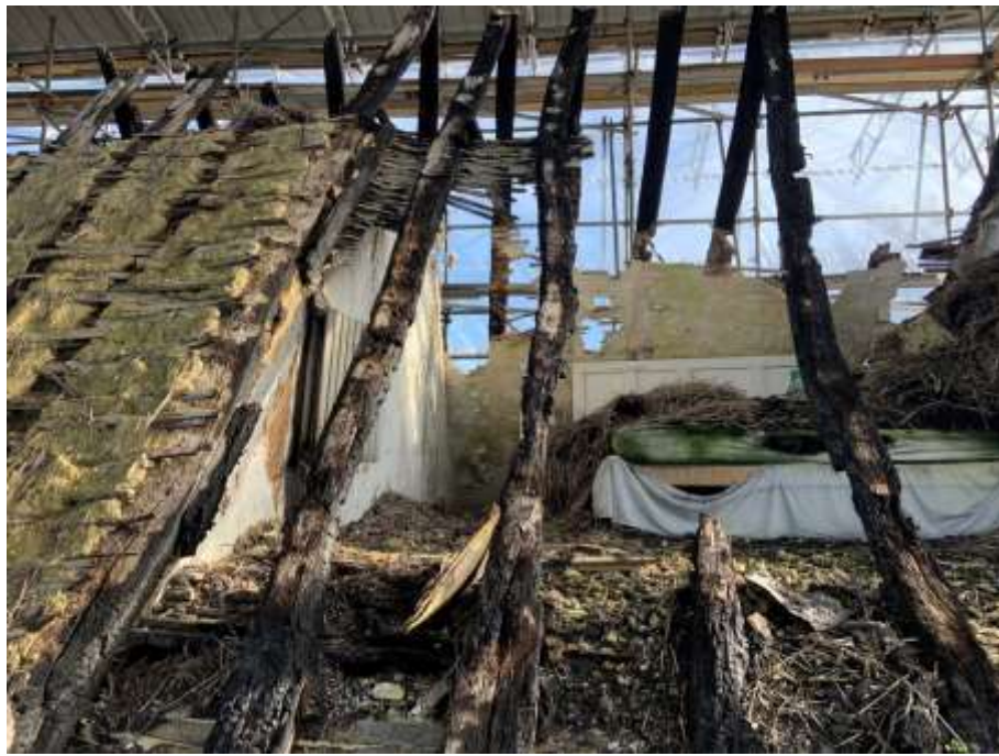
Plate 15. Roof 3 – Right-hand side upper level roof.
