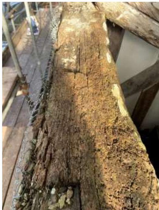
Plate 14. Wall plate at the front wall.
