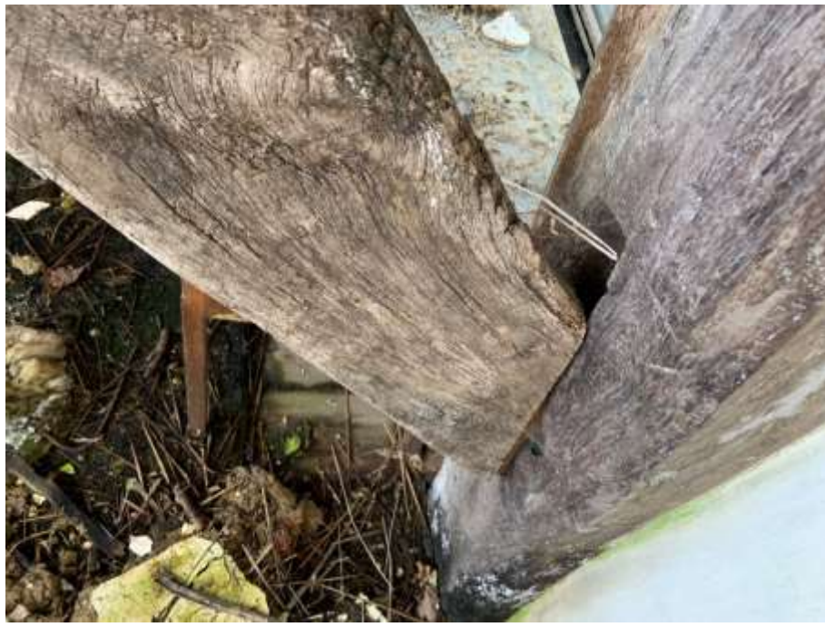
Plate 11. Gallows bracket to column connection.
