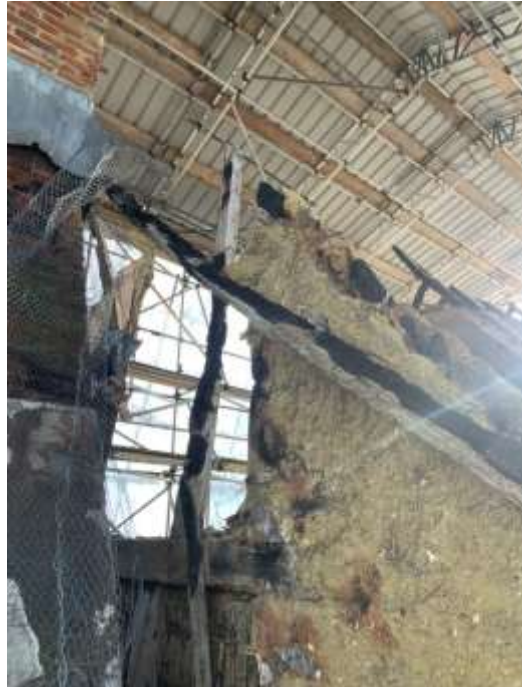
Plate 13. Timber framed, cob infill internal gable wall.
