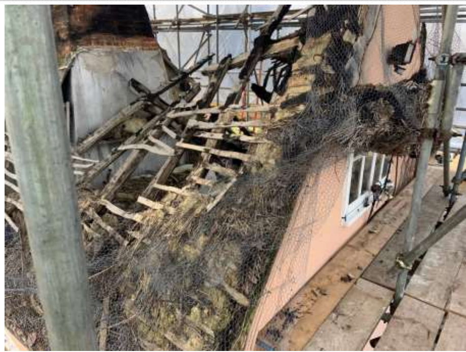
Plate 7. Back of Roof 1.
