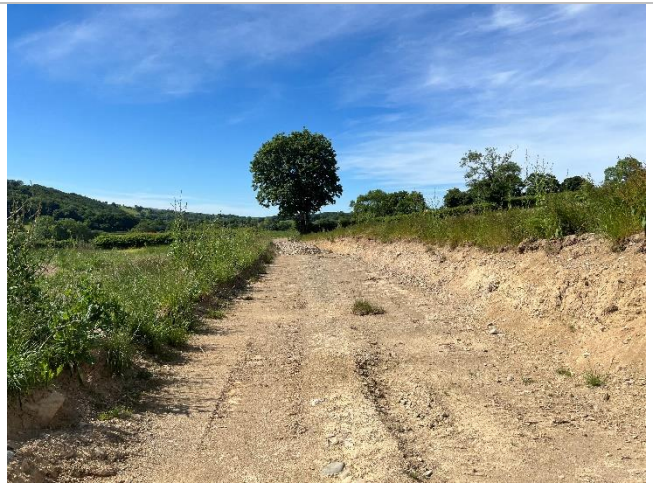
Existing access track.
