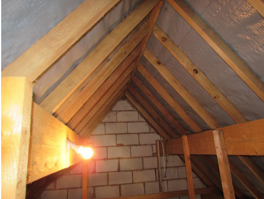
Plate 7 – Inside the east loft void
