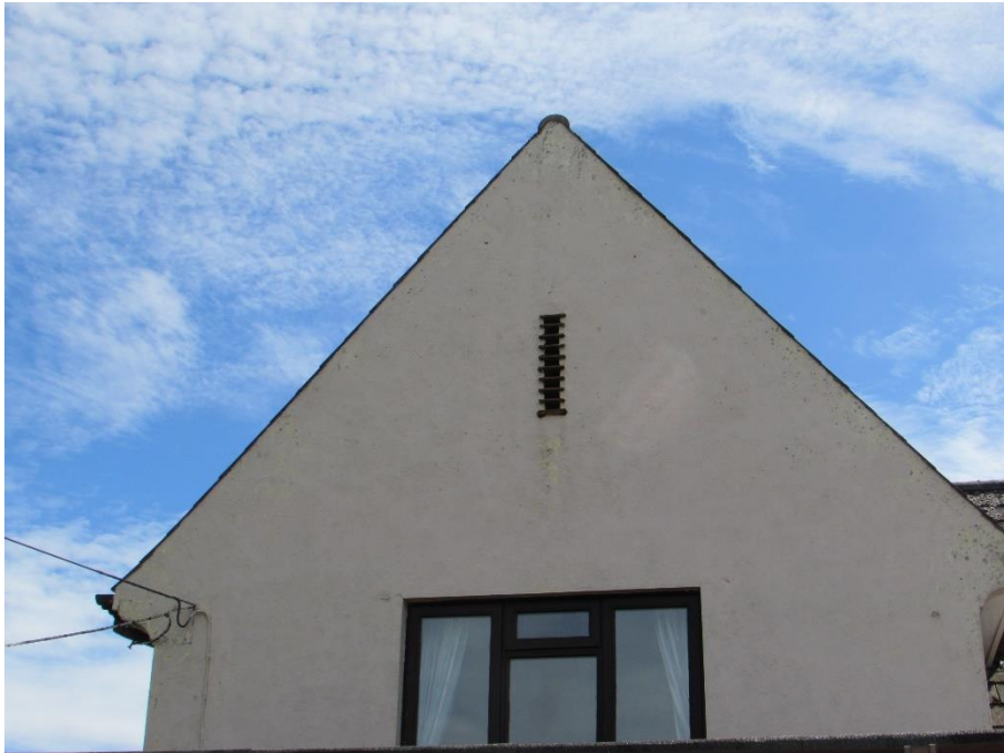
Plate 2 – The louver on the western elevation of the house
