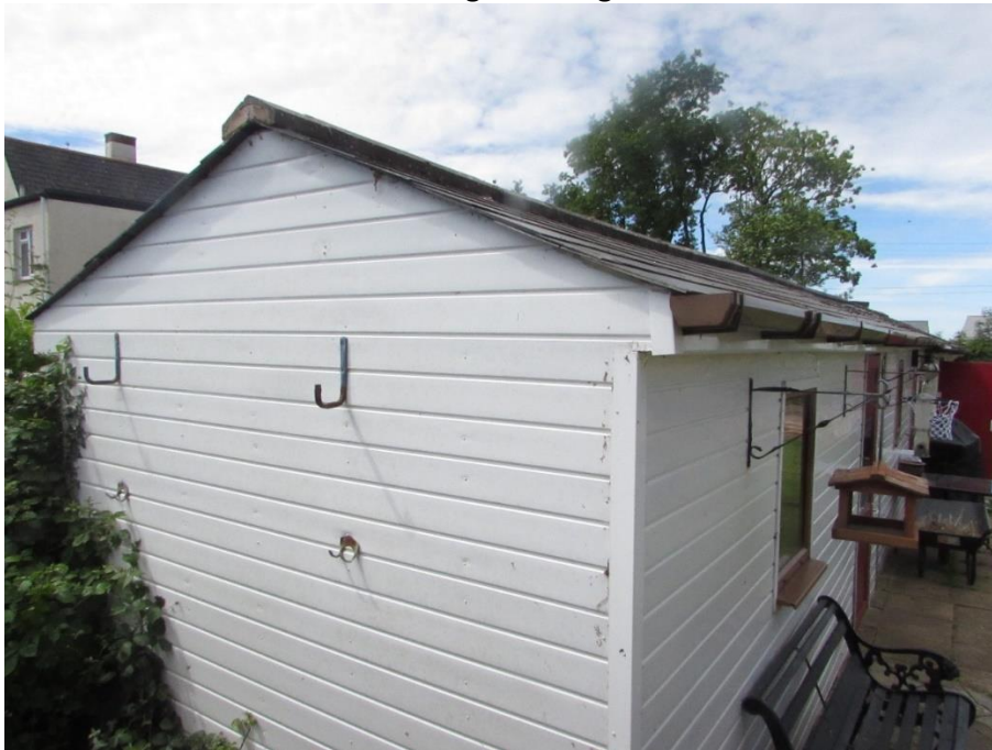
Plate 6- East elevation of the storage building
