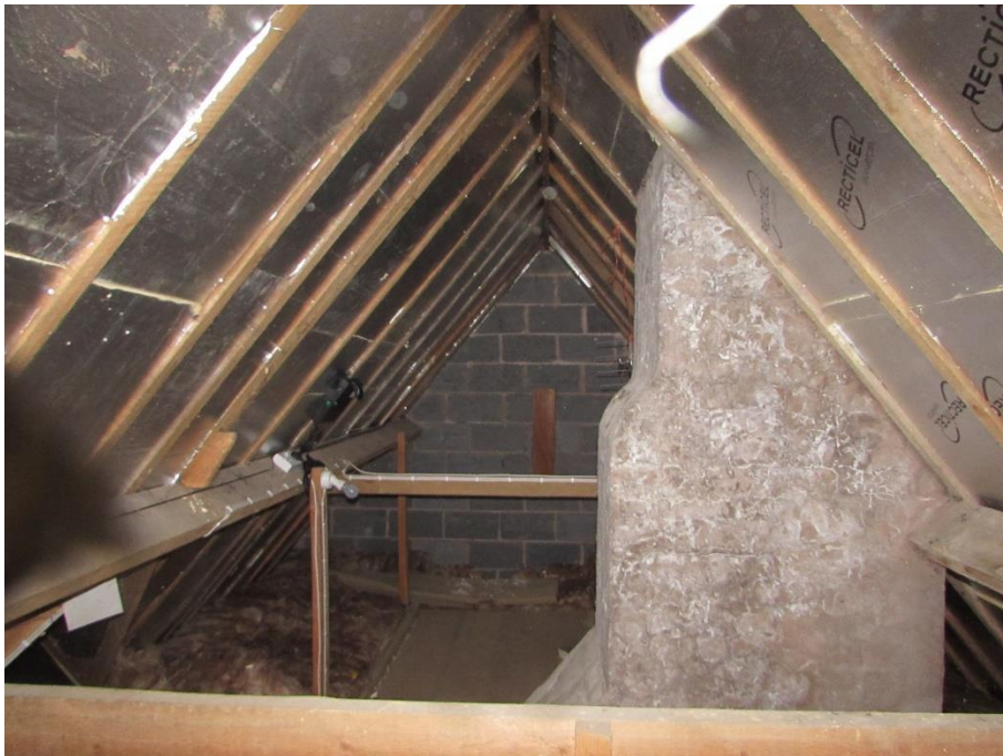
Plate 6 – Inside the west loft void
