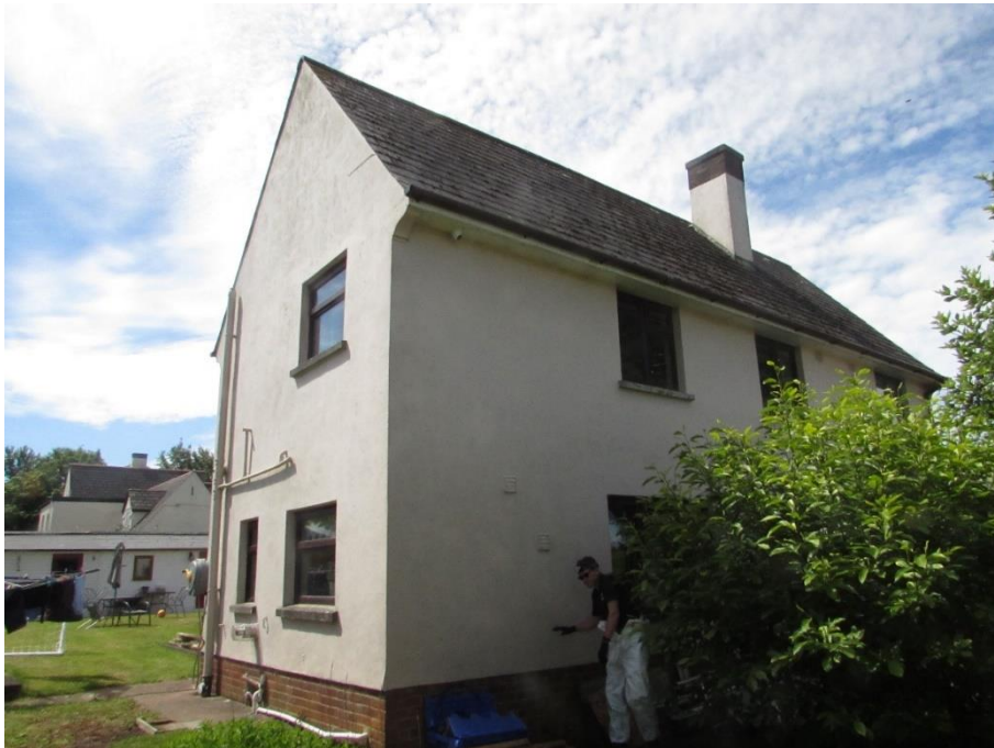
Plate 4 –North-east elevation of the house.
