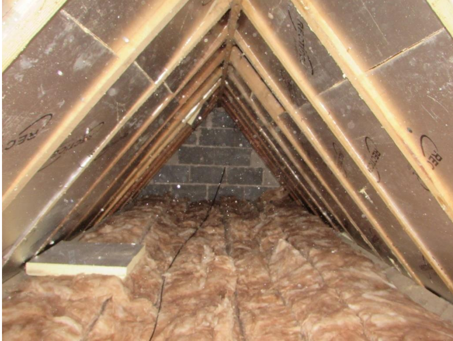
Plate 5 – Inside the south-west loft void
