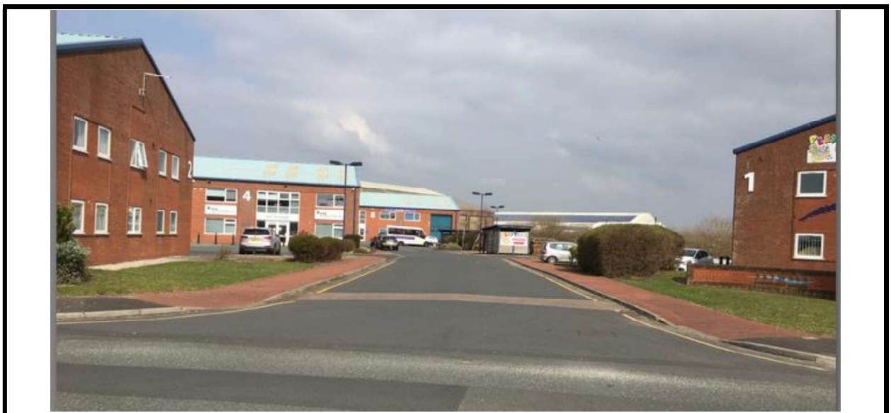
View to cul de sac leading to site access
