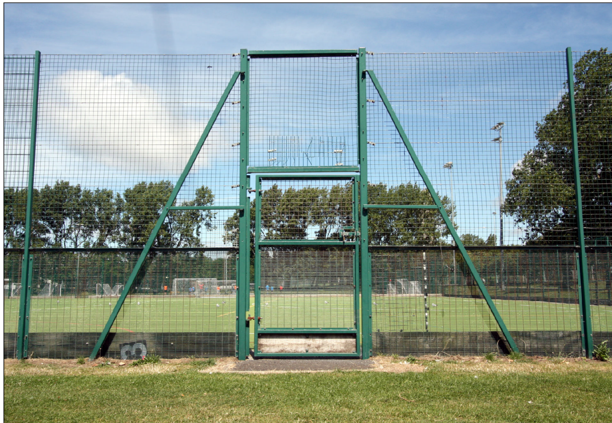
Plate 4) Gate and fence detail on current south elevation.
