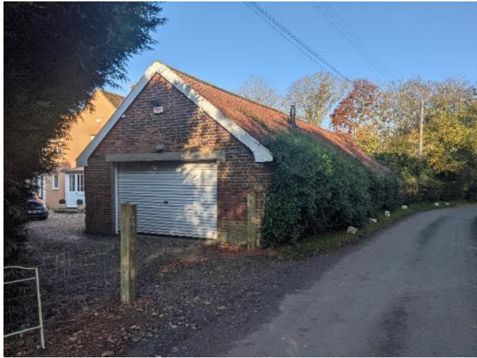
Photo 1 South and east elevation of garage and cart lodge
