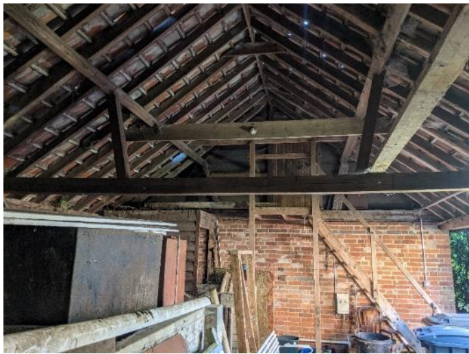
Photo 9 Internal view of the cart shed
