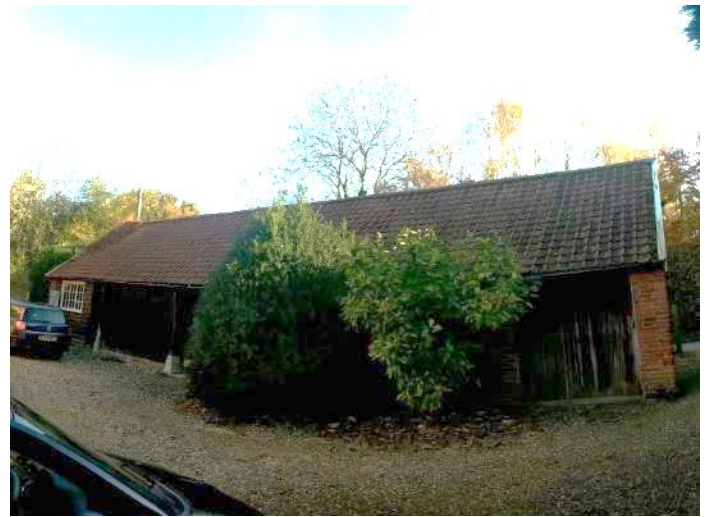
Photo 4 West elevation of garage and cart lodge – panoramic view
