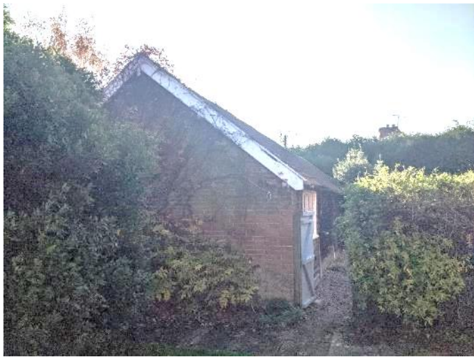
Photo 3 North gable end of cart lodge
