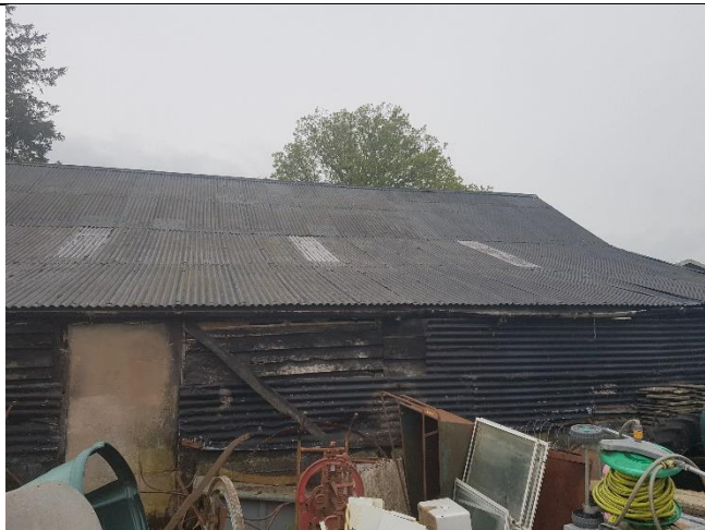
North east facing roof and lean-to.
