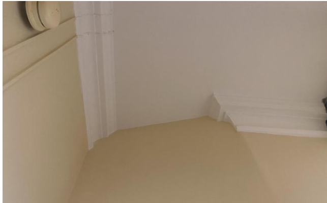
Existing disruptions to cornice indicating location of former partition
