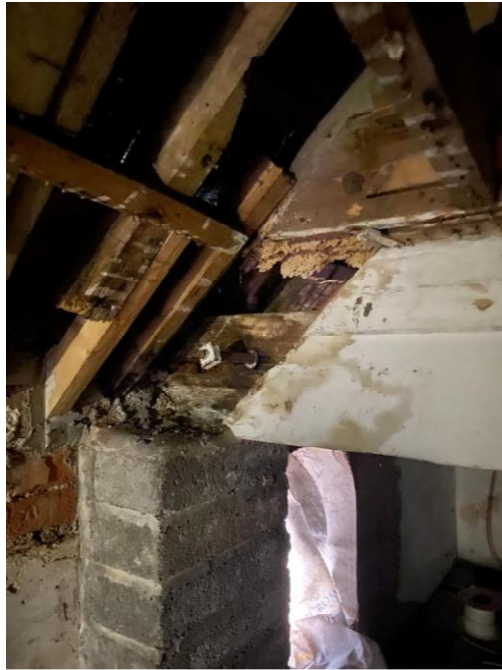
East truss foot
