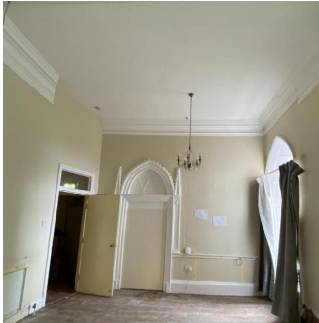
Existing disruptions to cornice indicating location of former partition
