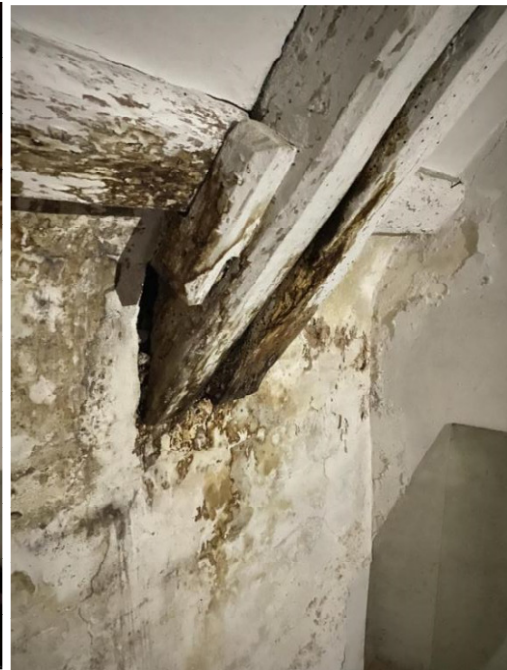
West truss foot
