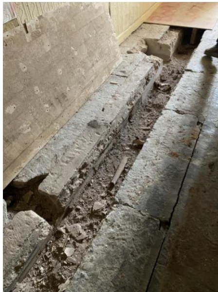
service trench with connections to G. 04
