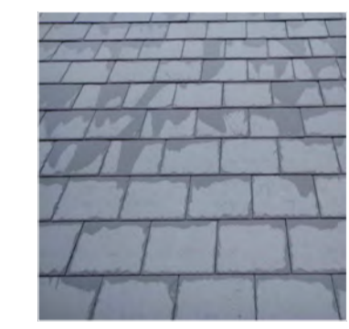
Spanish slate roof tiles (Main Roof)
