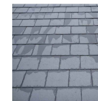
Spanish slate roof tiles (Main Roof)
