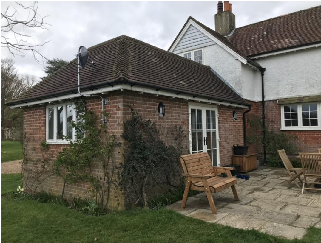
Figure 2. Part of existing west elevation showing later addition.
