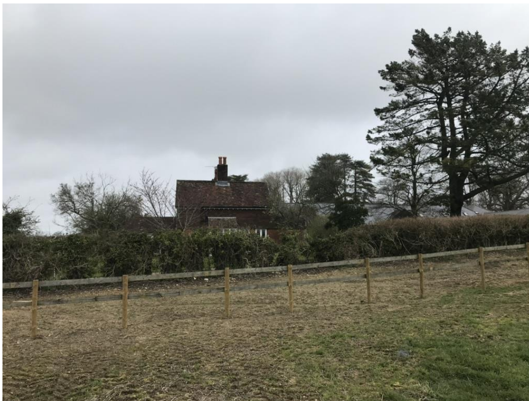
Figure 5. Contextual view of existing south elevation.
