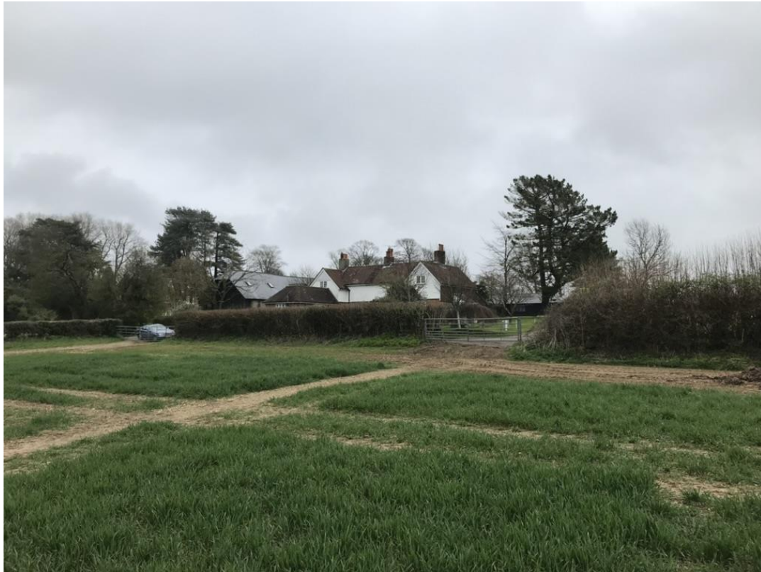
Figure 4. Contextual view of existing west elevation.
