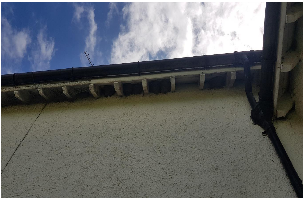
Picture 4: Showing the active House Martin nests on the western elevation
