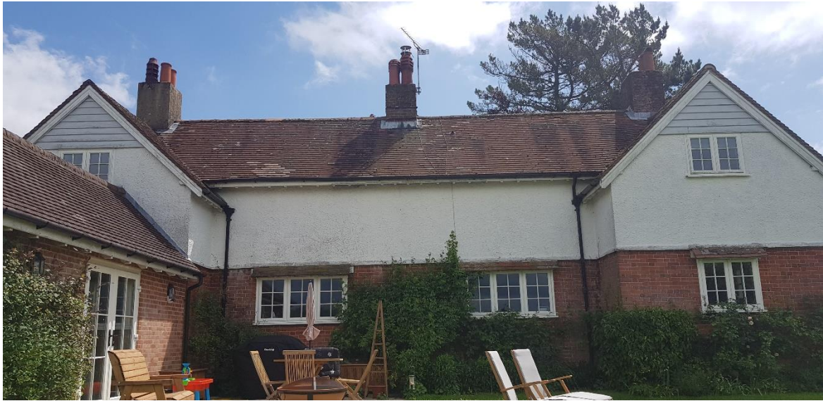
Picture 1: Showing the western elevation
