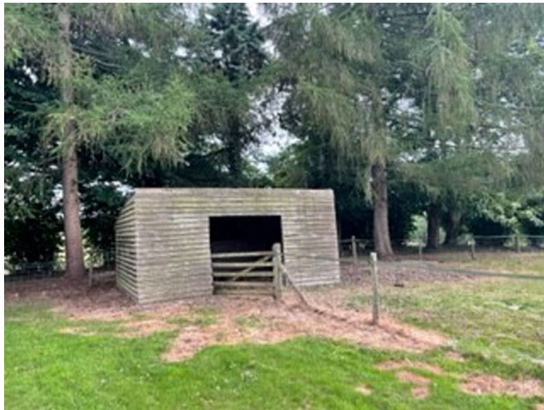
Fig. 3 – Existing field shelter frontage
