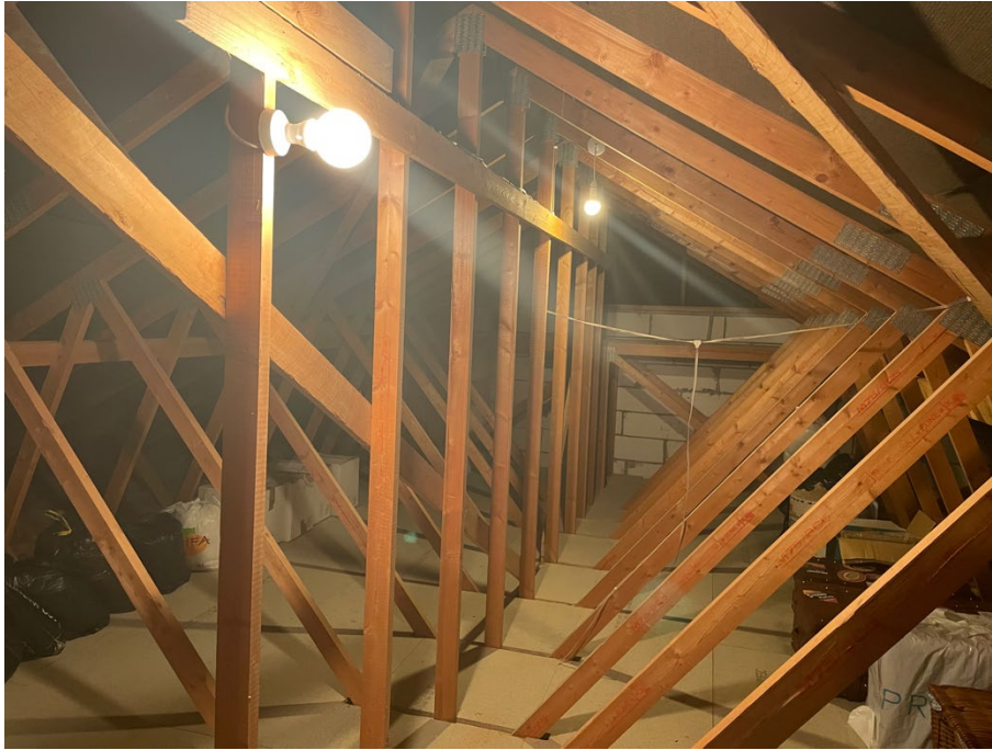
Photo 7: Roof void interior.
