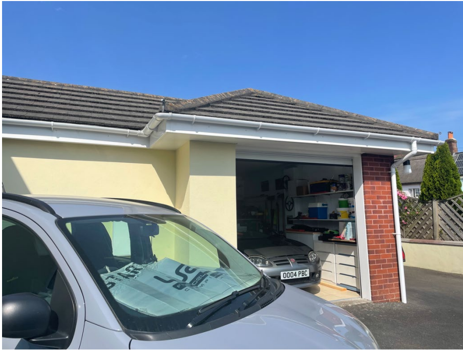
Photo 3: East elevation of garage.
