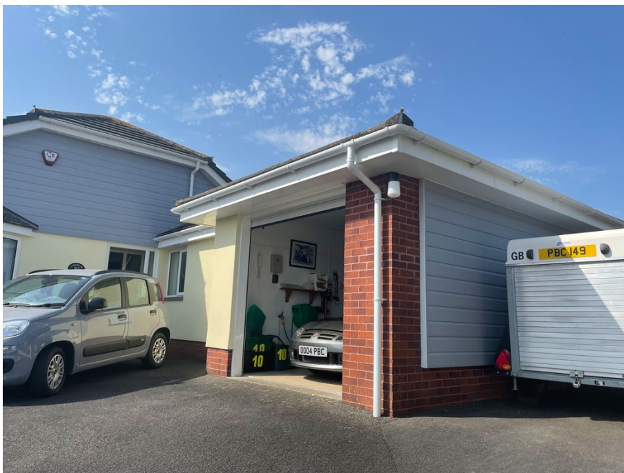
Photo 2: East and north elevations of garage.
