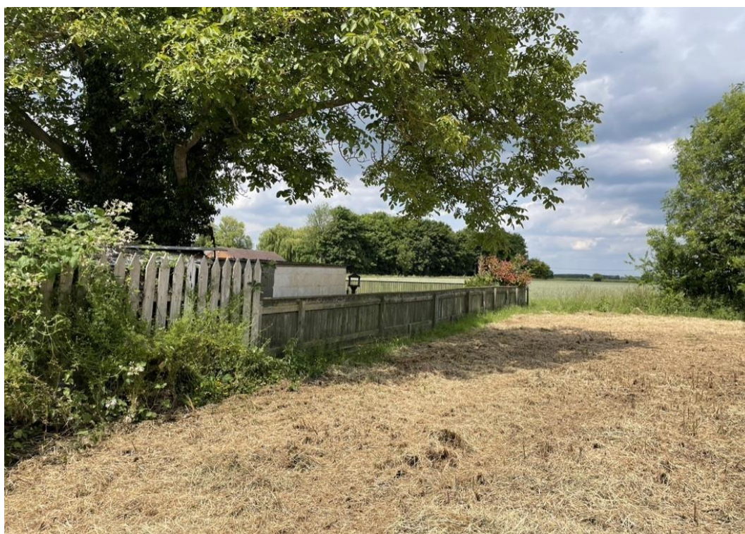
Photograph 15: Timber fencing which forms the northern end of the west boundary
