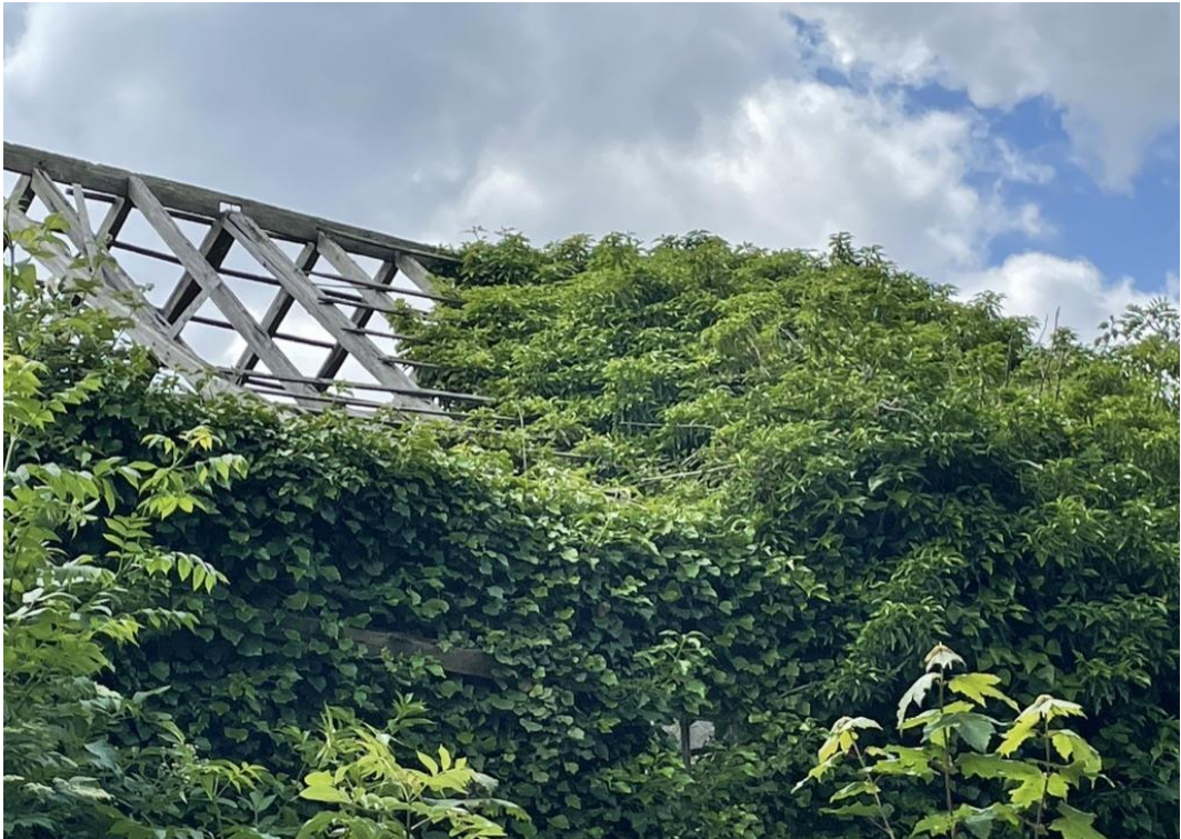
Photograph 8: Timber trusses and dense vegetation - building 2
