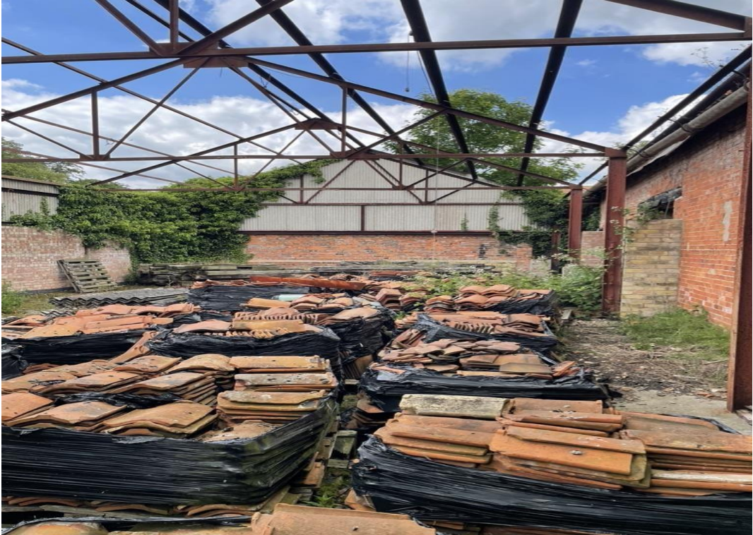
Photograph 7: Internal view of building 1
