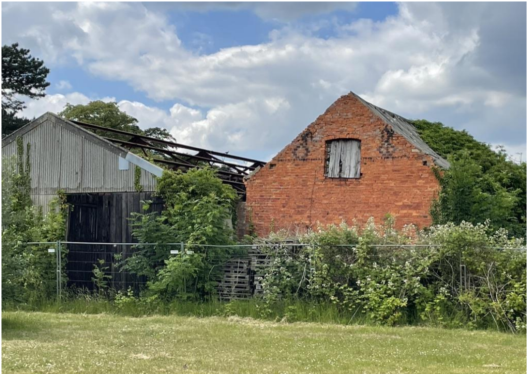
Photograph 9: Building 2 eastern elevation
