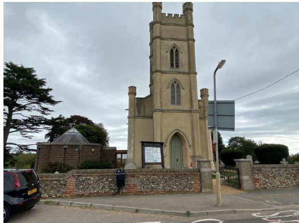
Fig 2. View of the Church of St Mary's and All Saints from Church Road.
