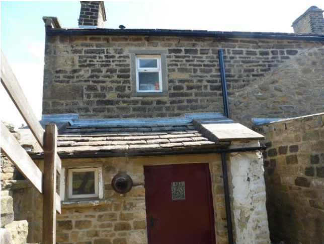
Existing house (rear elevation Shared Alleyway)
