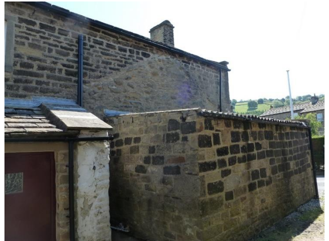
Existing house (rear elevation Shared Alleyway)
