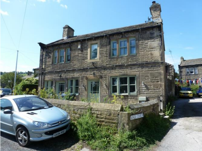
Existing house (front elevation High Street)
