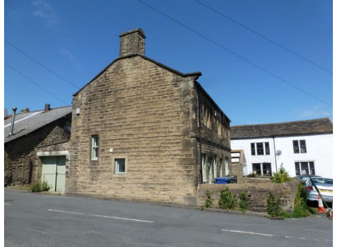
Existing house (side elevation West Lane)
