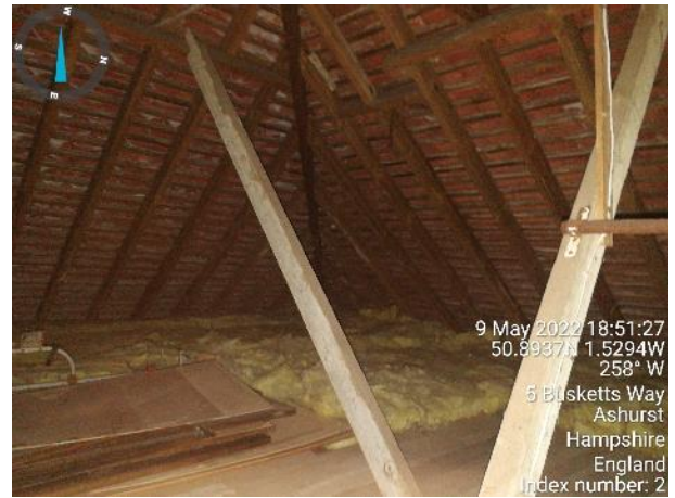
Photograph 2: View of interior of loft.
