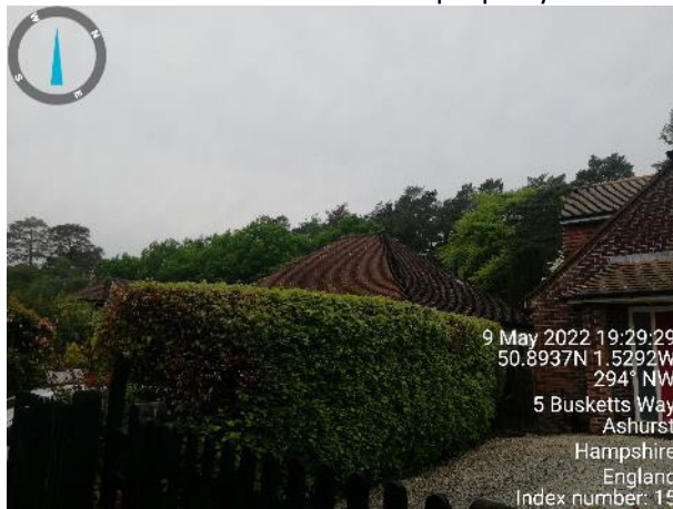
Photograph 13: View of the east section of hipped roof from the road.
