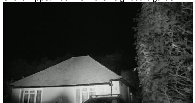
Photograph 16: View of the front of the property with the NVA's 09/05/2022.
