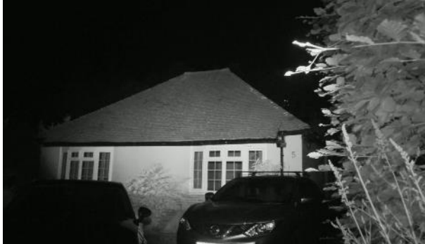
Photograph 19: View of the front of the property with the NVA's 09/06/2022.
