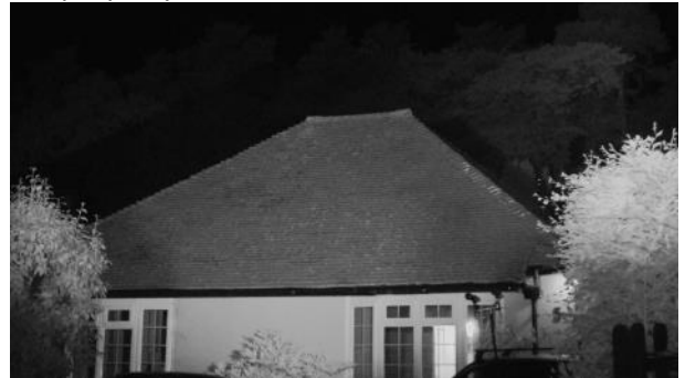
Photograph 22: View of the front of the property with the NVA's 23/06/2022.
