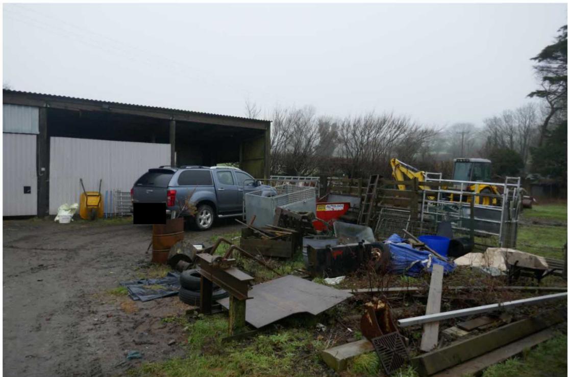
➤ Photograph looking the front elevation of the existing barn.
