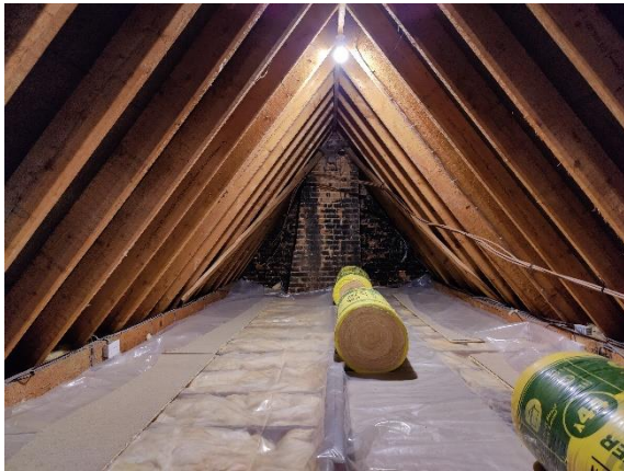
Photo 5 Interior of loft – north end showing modern roof timbers and new plastic sheets
