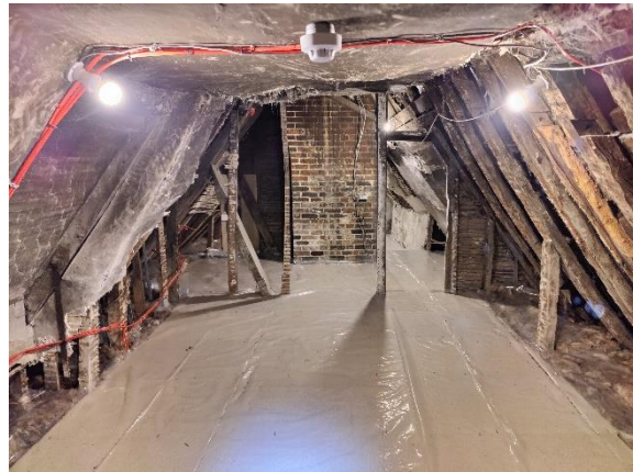
Photo 6 Interior of loft – south end showing brick chimney and new sheeting
