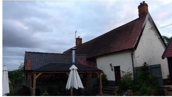
Photo 2 North east elevation (rear) showing beer garden
