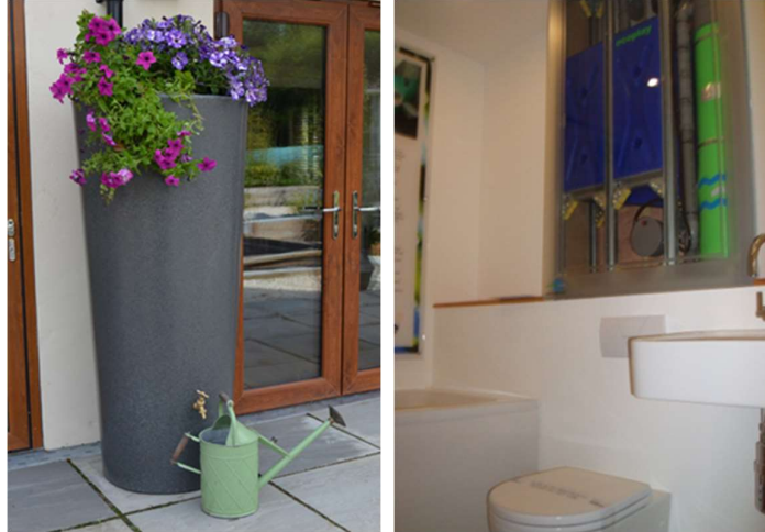
Figures 7 & 8: External rainwater harvesting butt & EcoPlay unit above WC
