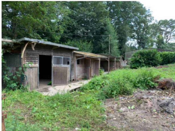
Figure 11: North-west elevation of existing barn
