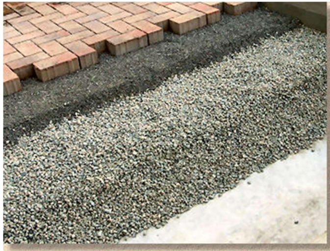
Figure 9: Typical permeable paving solution
