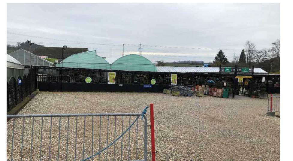
Figure V - View of polytunnels currently on site.
