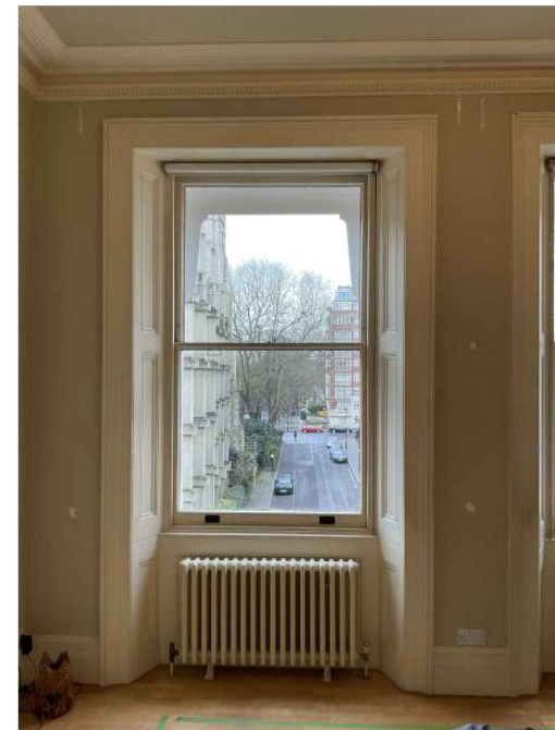
EXISTING W01 ON SECOND FLOOR
