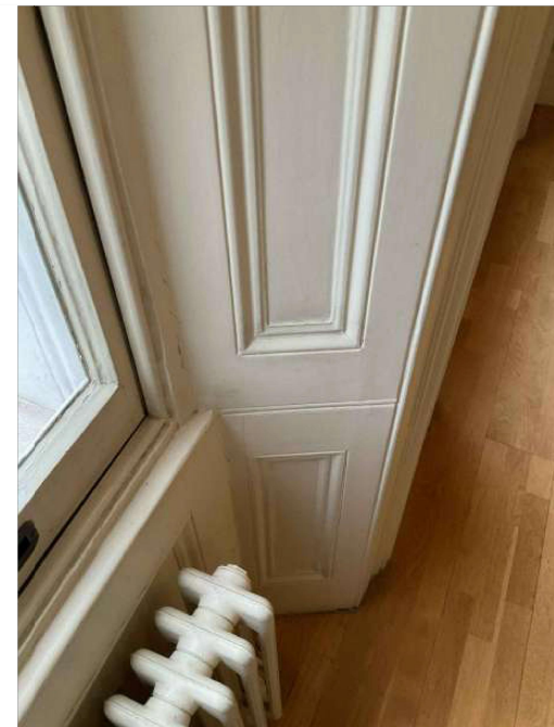
EXISTING W01 ON SECOND FLOOR
