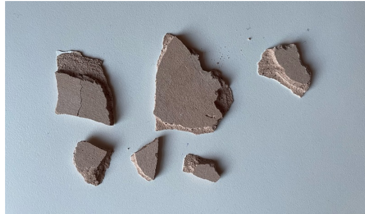
Figure 11: Existing Ceiling Material Assumed to Comprise Contemporary Multi-Finish Plaster
