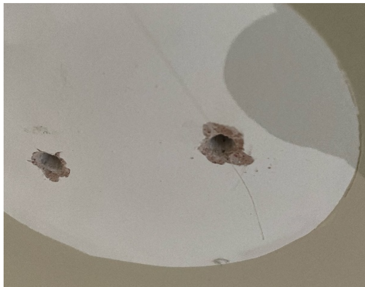
Figure 9: Guest Bedroom Existing Ceiling
