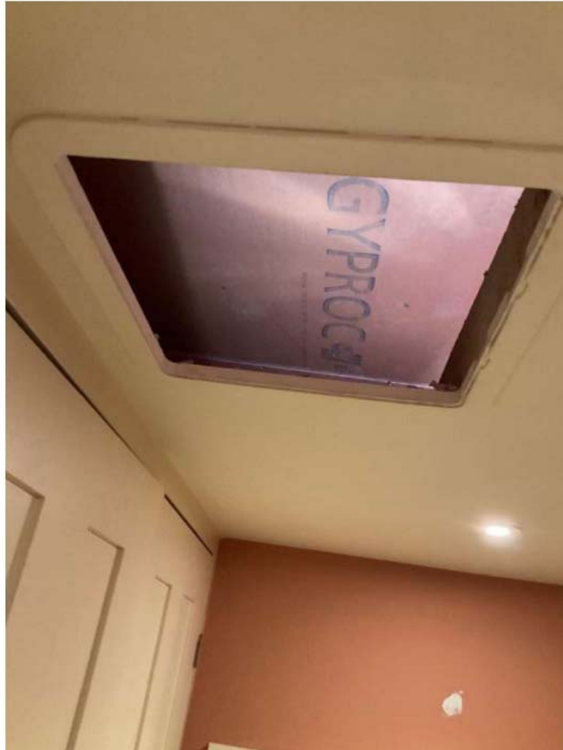
Picture 8: Existing secondary ceiling halls and bathroom areas
