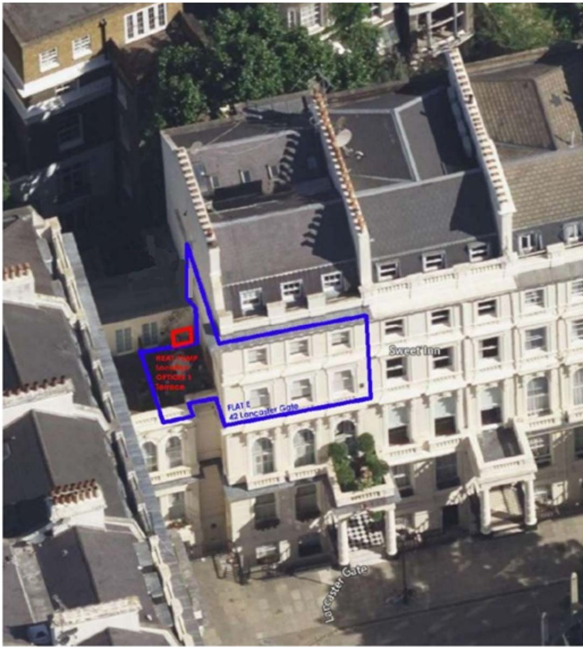
Picture 1: Location for the installation of the external heat pump condenser.
