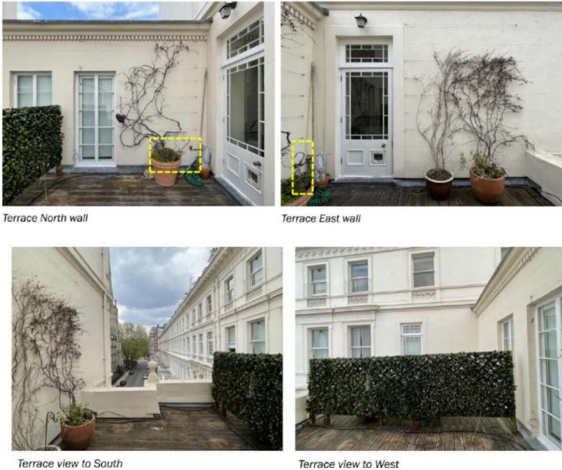
Picture 2: Terrace installation and positioning of outdoor unit.
