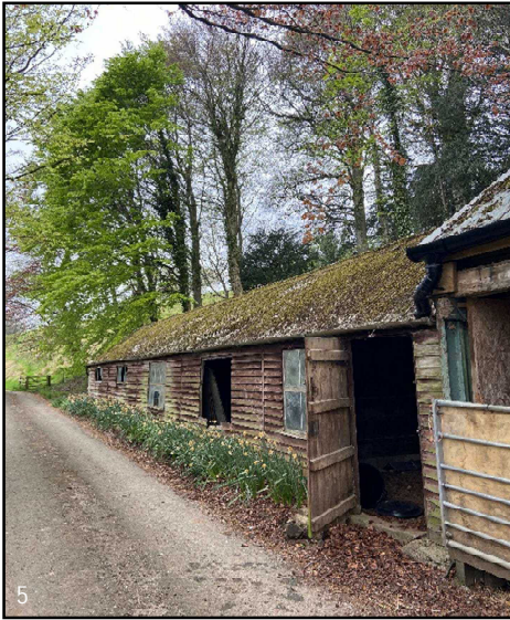
Plate 5. View of the south-east corner of the barn
