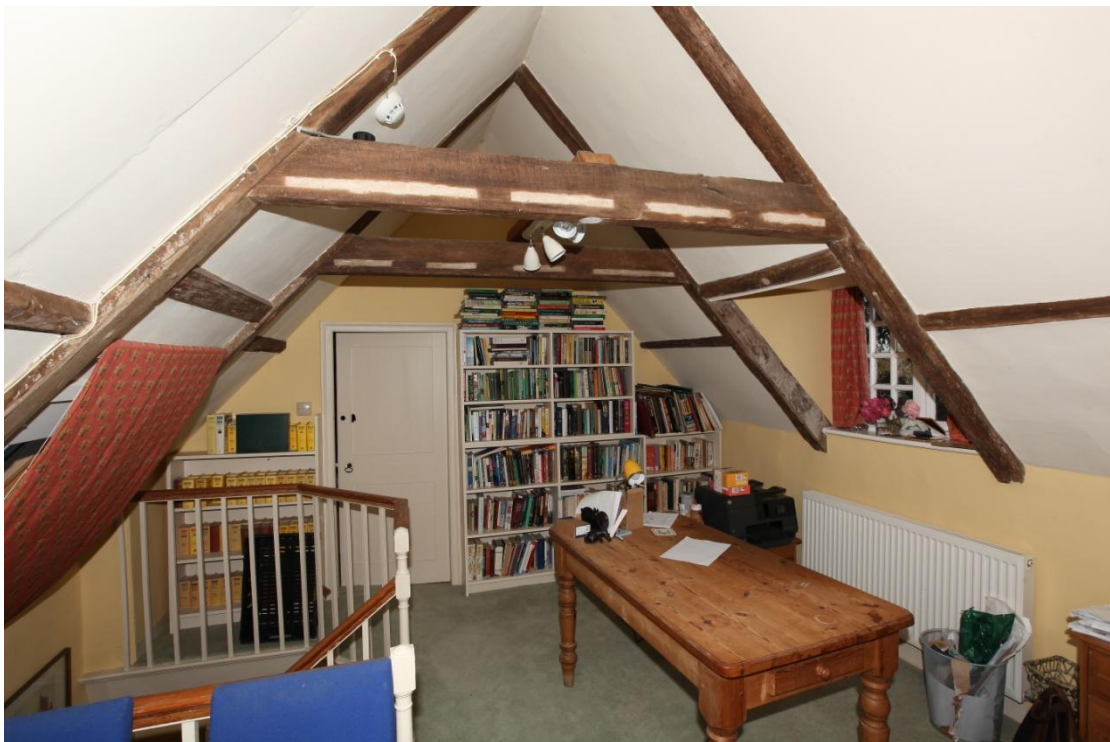
Illus. 34. The roof of the Georgian range, as seen from the west with the staircase to the left. The staggered butt-purlins are clearly original, respecting the positions of the southern dormer windows, but the collars appear to have been re-used and contain wide plaster-filled mortices in their western edges and smaller joist mortices to the east.
