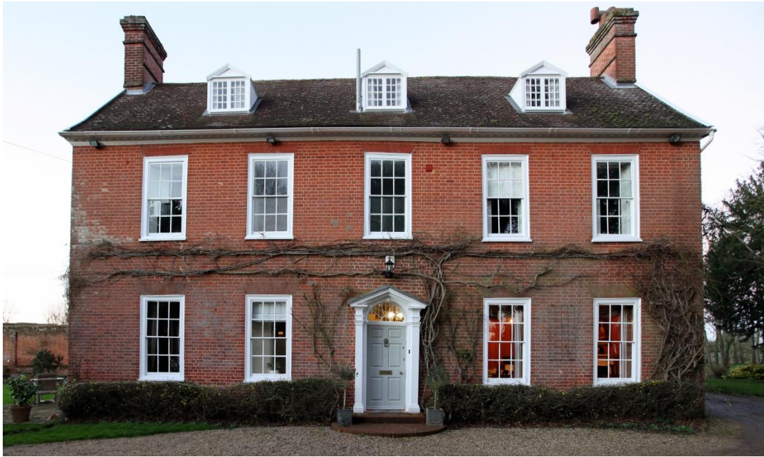
Illus. 1. The handsome, symmetrical late-Georgian southern facade, which remains unaltered since it was built – probably by William Ray the Younger who owned the property between 1768 and his death in 1790.
