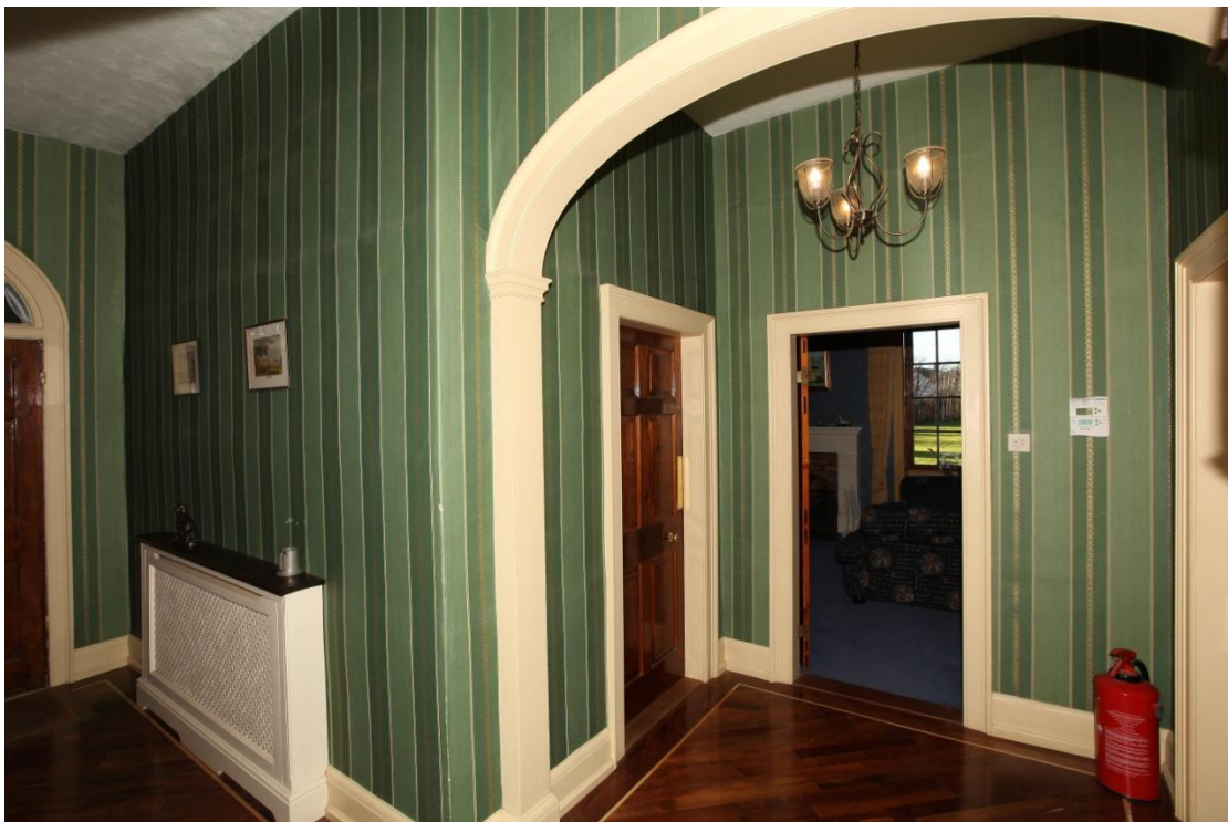
Illus. 28. The arched lobby to the west of the Georgian entrance passage, with the door to the 16 th century hall on the right. This unusual feature was necessary to reach the approximate position of the Tudor cross-passage and partly replicates the porch shown in figure 4 – although there is nothing to suggest any of its fabric survives. The partition to the left is original and the central door opens into the modern ‘sitting room’. If the left-hand WC door existed initially it may have served a cupboard or butler’s pantry.
