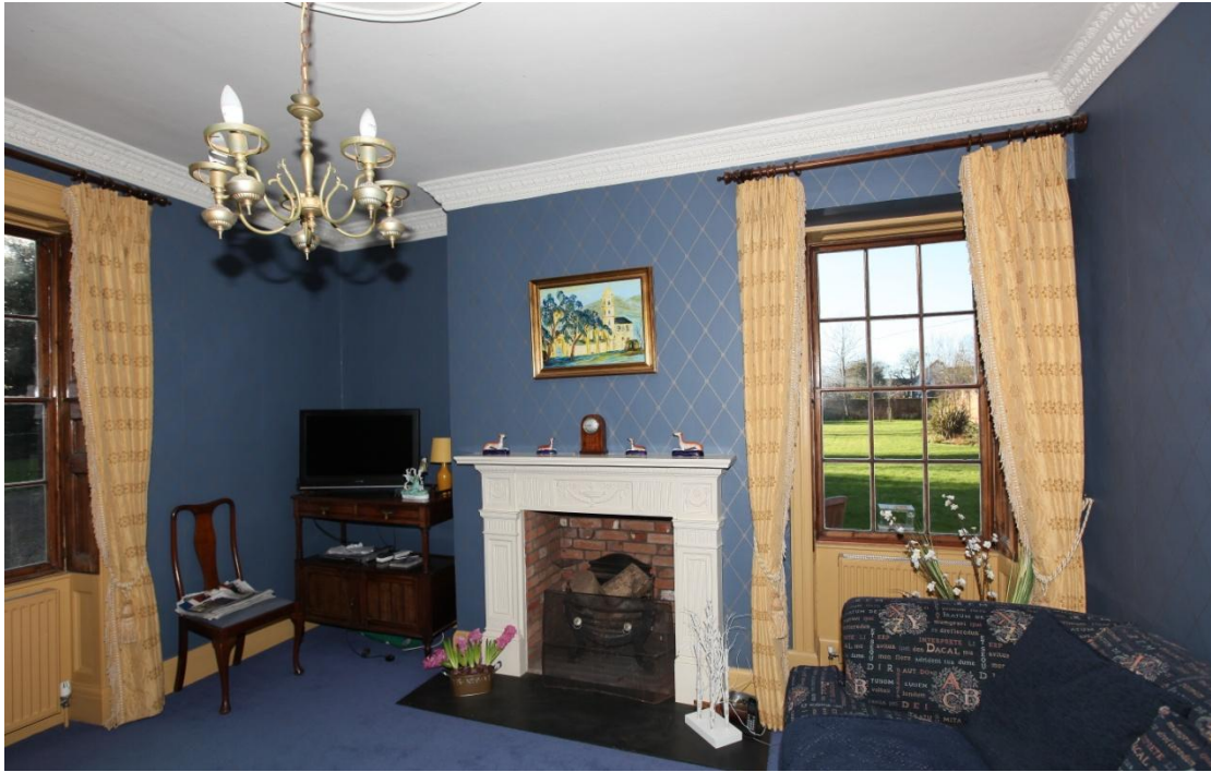
Illus. 29. The fireplace in the western gable of the Georgian ‘sitting room’. The exposed brickwork is modern and the carved fire surround appears to be a copy of an Adam-style original that matches the example in the dining room (illus. 31). The suspiciously sharp cornices of both rooms are also identical, in a way that would not be expected in the 18 th century. They are far more elaborate than would be expected in a house of this scale and in conjunction with the relatively plain but clearly original staircase. It would appear that a former owner installed these features as part of a major refurbishment.
