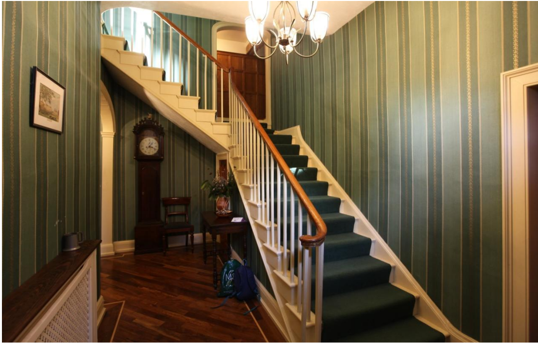
Illus. 27. The Georgian entrance passage from the southern front door, with the arched entrance to the Tudor building on the half landing. The elegant staircase is a fine original feature which rises to the attic storey but is relatively plain with a pine hand rail and no carving to the tread-ends.
