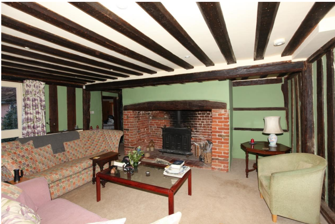
Illus. 8. The early-16 th century hall (the living room in figure 15) looking east towards the narrow high-end chimney bay of 1.4 m (4.75 ft) that was probably designed for a single, large fireplace heating the hall but not the parlour. The present fireplace is a reconstruction of the 18 th century, and the original brickwork would have adjoined the jambs of doors to the right and left that opened into the parlour and either a cupboard or newel stair respectively. The common joists of this room were hidden by lath-and-plaster as recently as 1997.
