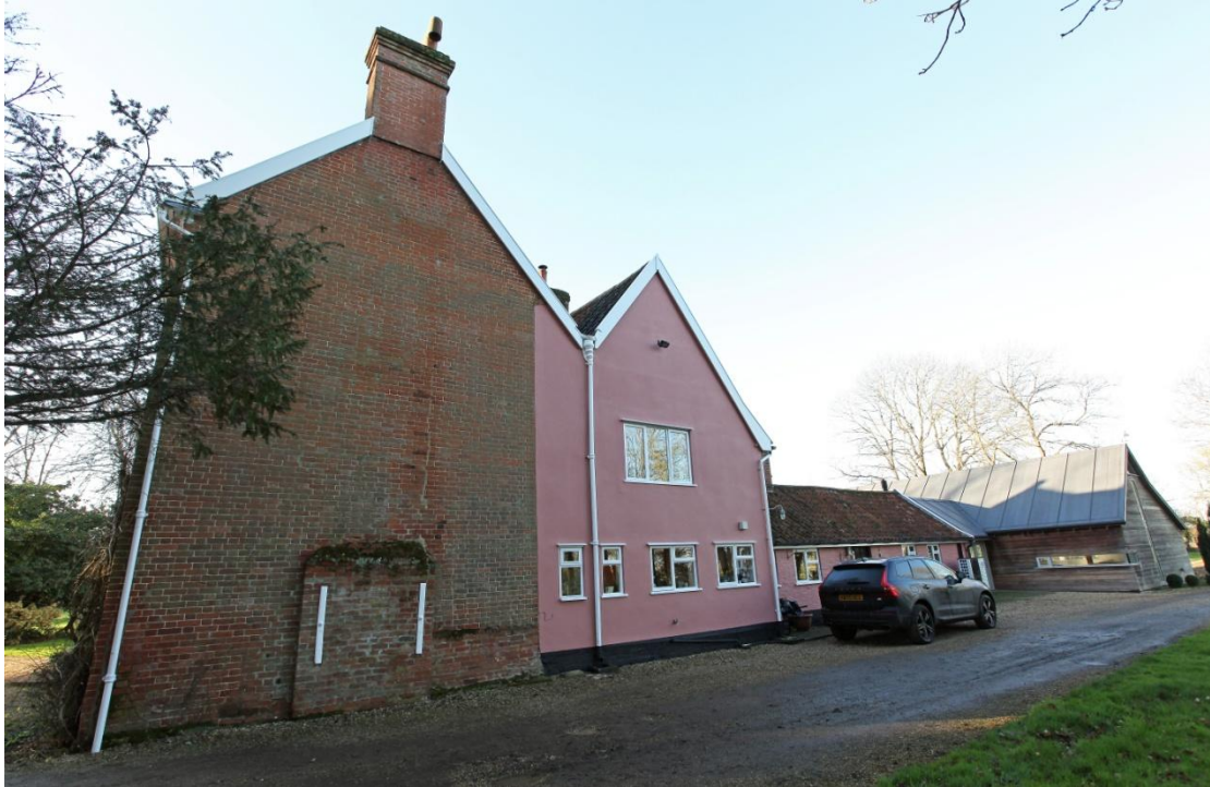
Illus. 3. The eastern gable was not visible from either the maltings or the road and was not disguised in the manner of its counterpart to the west. The rafters of the Georgian front range over lap those of the lower Tudor building giving the earlier gable a false appearance of asymmetry.
