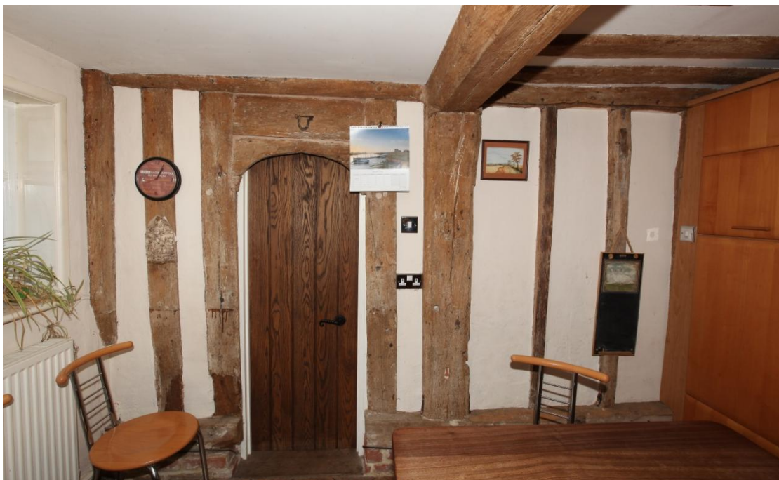
Illus. 12. The front wall of the two-bay parlour (now the kitchen), showing an original arched door to the left and the shutter groove and mullion pegs of a window to the right. Separate parlour entrances became increasingly common as the 16 th century progressed but this example is unusually early. It may have been intended to access the adjacent outbuilding shown on early maps.
