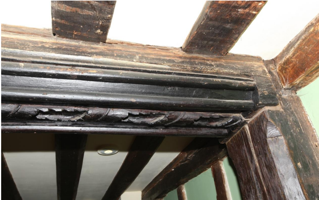
Illus. 11. A detail from the low-end bay of the finely roll-moulded binding joist in the hall, with a foliate-carved scroll to the centre of its soffit. This timber is fully pegged and tenoned to the storey posts and undoubtedly original to the building, although it is unusual to find roll-mouldings of this kind in conjunction with plainly chamfered and unchamfered common joists. The foliate scroll is typical of the 1520s but is crudely carved compared with identical examples found in many merchant houses and churches of the period.
