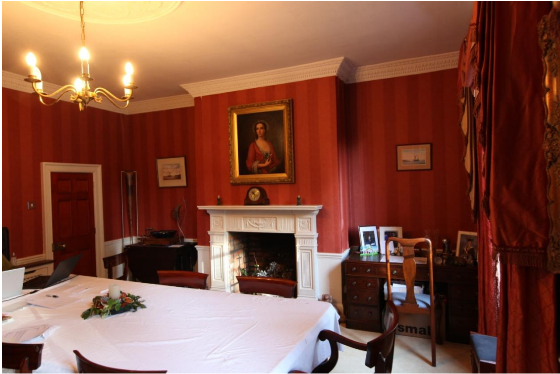
Illus. 31. The eastern gable of the Georgian ‘dining room’, with the arched entrance of the Tudor parlour in illustration 13 hidden behind the door on the left. As in the ‘sitting room’, the fireplace, cornice and plaster ceiling rose appear to be late-20 th century insertions. The principal drawing and dining rooms of Georgian houses were rarely decorated in the same way, with the better quality ornament reserved for the latter.
