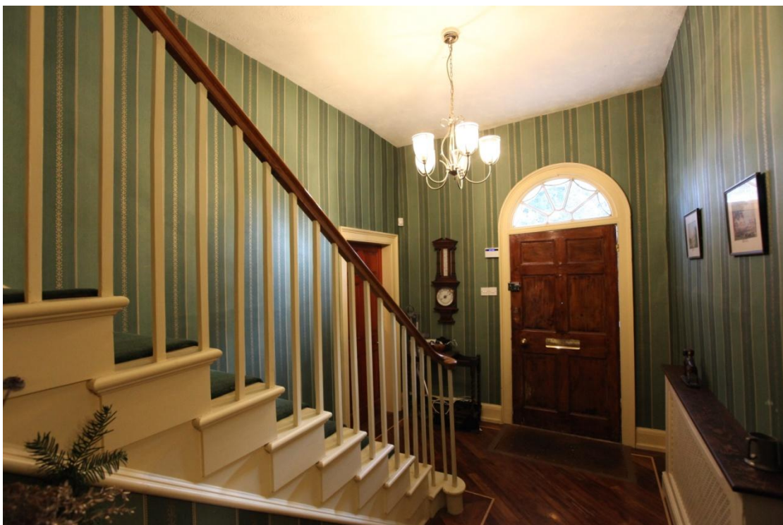
Illus. 26. The central entrance passage of the Georgian addition which retains its original 'stick' baluster staircase and fanlight. The door is slightly offset as usual to accommodate the foot of the stair, and this arrangement is fully original to the building.
