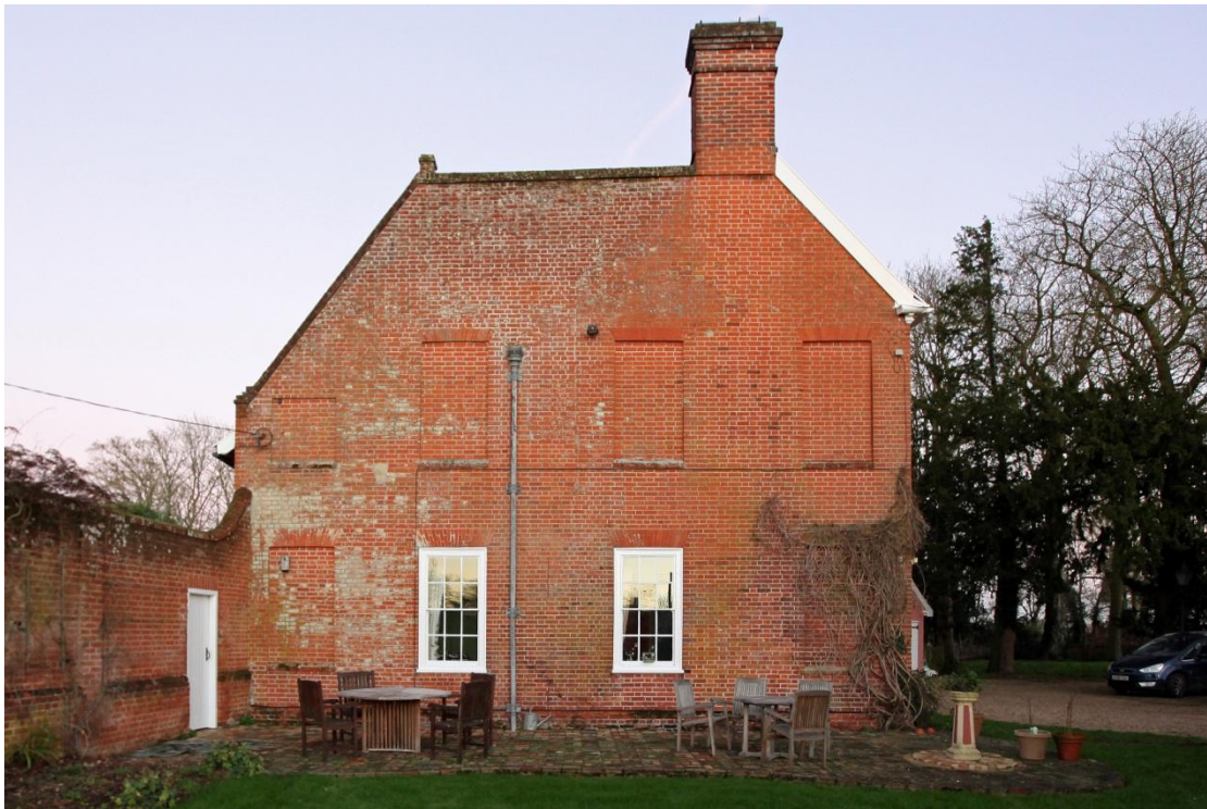
Illus. 2. The remarkable Georgian western gable which disguises the earlier timber-framed structure to the left. Its blind windows were designed as such, and were intended to relieve the considerable expanse of brickwork. They bear no relationship to the Tudor building, and it was necessary to raise the ceiling in the latter's service bay in order to accommodate the ground-floor window to the left. Both first-floor windows to the left of the drain pipe are obstructed by the original tie-beam in illustration 23.
