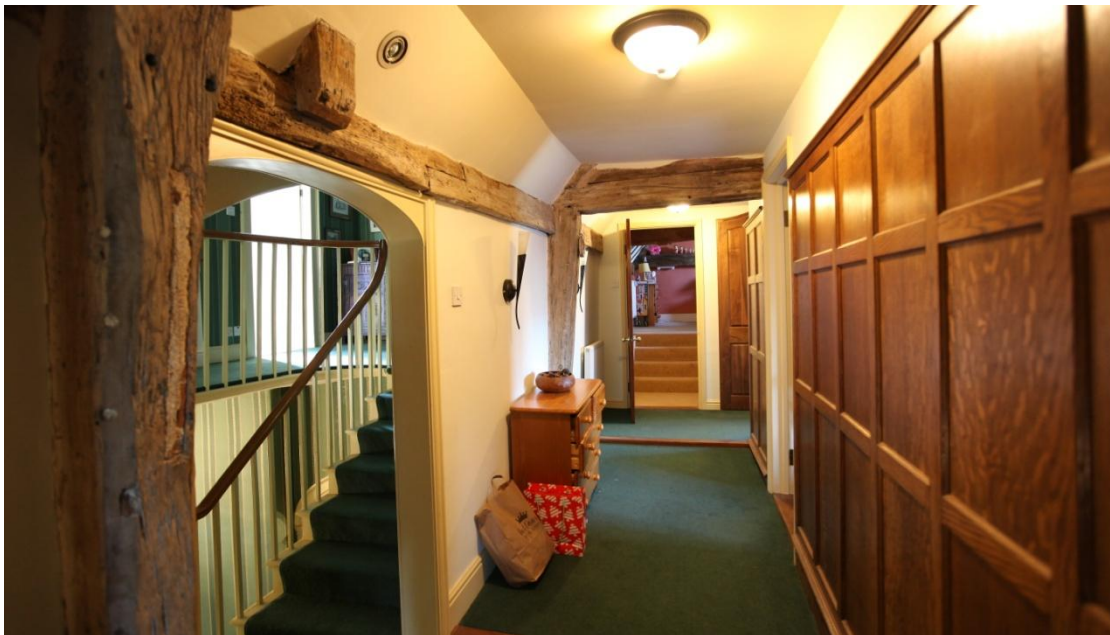
Illus. 16. The first-floor corridor to the south of the hall chamber, as seen from the chimney bay to the east, with the Georgian staircase to the left. Note the steps leading to the service chamber in the rear (bedroom 3), which was raised to accommodate the Georgian window of the western gable. The panelling is modern.
