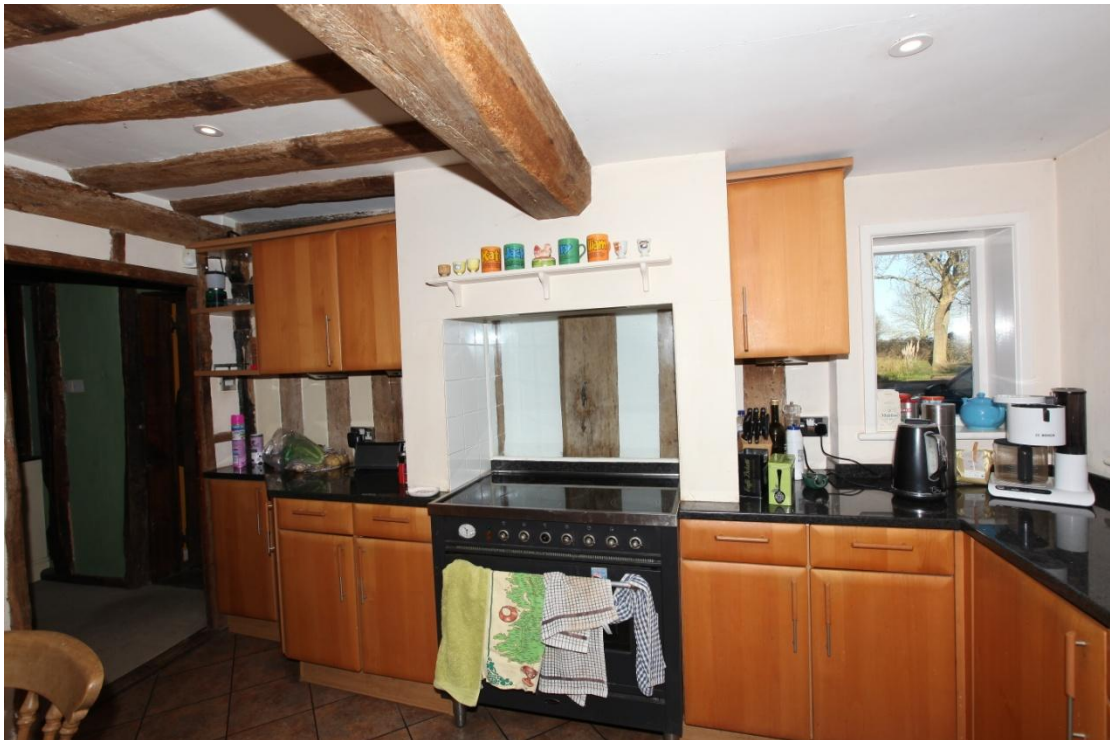
Illus. 14. The rear (northern) wall of the parlour with the position of the original window in illustration 15 to the left of the binding joist. The exposed common joists are chamfered like those in the high-end bay of the hall but it is unclear whether they survive above the modern dry-lining which conceals the eastern bay on the right. The gable is also dry-lined with what appears to be plasterboard at this level, and may have been rebuilt.
