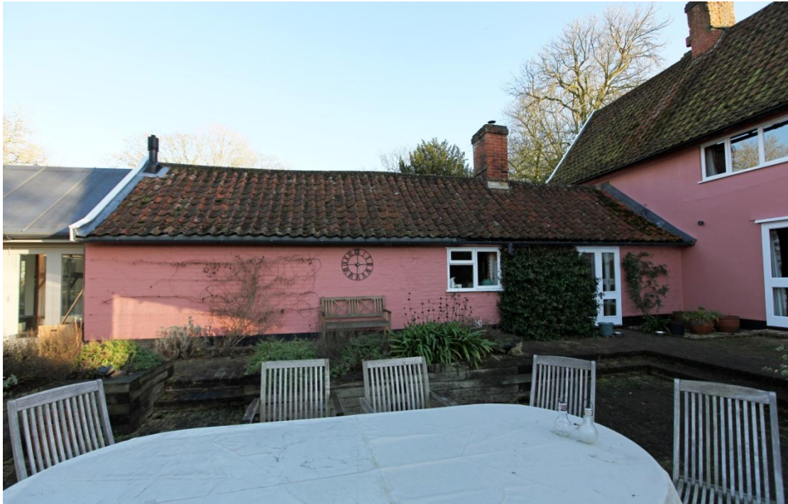
Illus. 5. The brick rear service range from the west with the Tudor house on the right and the addition of 2011 which forms part of the covered swimming pool on the left. The chimney was roughly central to the original structure as shown in figure 12, but it had been extended to its present length by the 1970s. The swimming pool of circa 2000 extended from the clock to the northern gable on the left and the new brickwork that filled the wide connecting door is visible to the left of the bench. This rear yard lies in the expected position of the medieval house at the centre of the moat.
