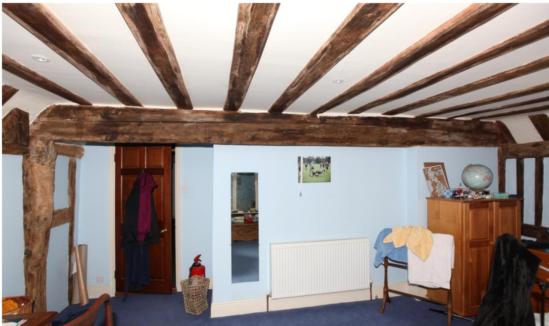
Illus. 22. The tie-beam to the west of the parlour chamber (bedroom 1). This abuts the chimney bay but there is no evidence of a fireplace in this room. The tie contains an unusual variety of pegged mortices, possibly for an arched doorway on the left which provided a link with the hall chamber (lit by the window adjoining the post to the left) and a gap framed by an arch-brace to the right of a central stud that would have exposed the chimney flue.
