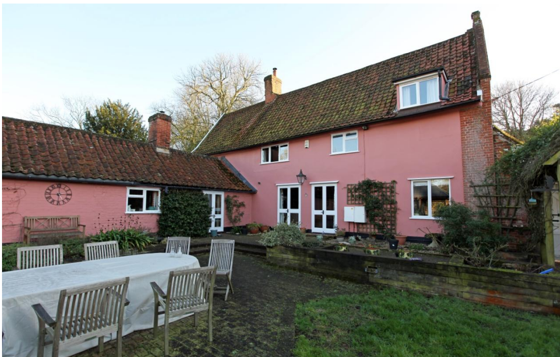
Illus. 6. The rear (northern) elevation of the early-16 th century house with the brick western gable in illustration 2 on the right. The windows date from a major late-20 th century refurbishment which occurred prior to 1997. Figure 12 shows small-paned casements that may have survived from the Georgian remodelling.
