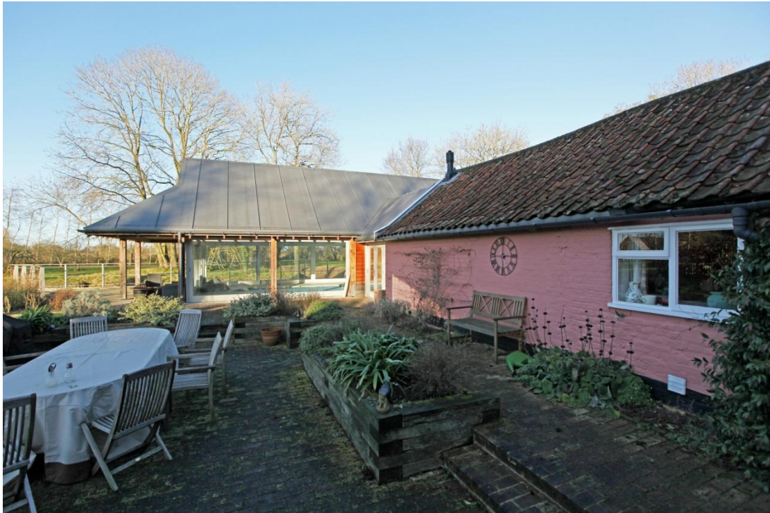
Illus. 7. The rear courtyard from the south showing the covered swimming pool of 2011 adjoining the single-storied service range.
