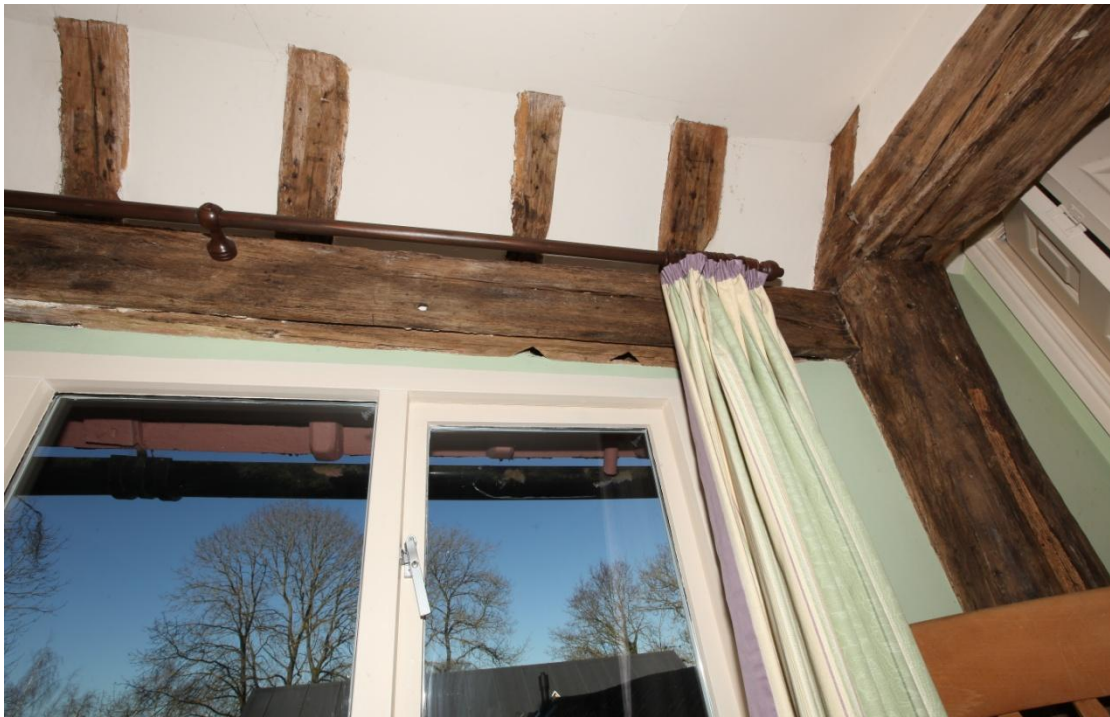
Illus. 18. A detail of the hall chamber's roof-plate in illus. 17 showing empty mortices for diamond window mullions, i.e. square mullions set diagonally in the standard manner of early unglazed windows. These illustrate the utilitarian nature of the space relative to the adjoining parlour chamber which boasts chamfered mullions. Impressive as the roof structure might appear, it was visible from this space and was probably regarded as practical rather than decorative: hall chambers were typically store rooms while parlour chambers were secondary bedrooms.
