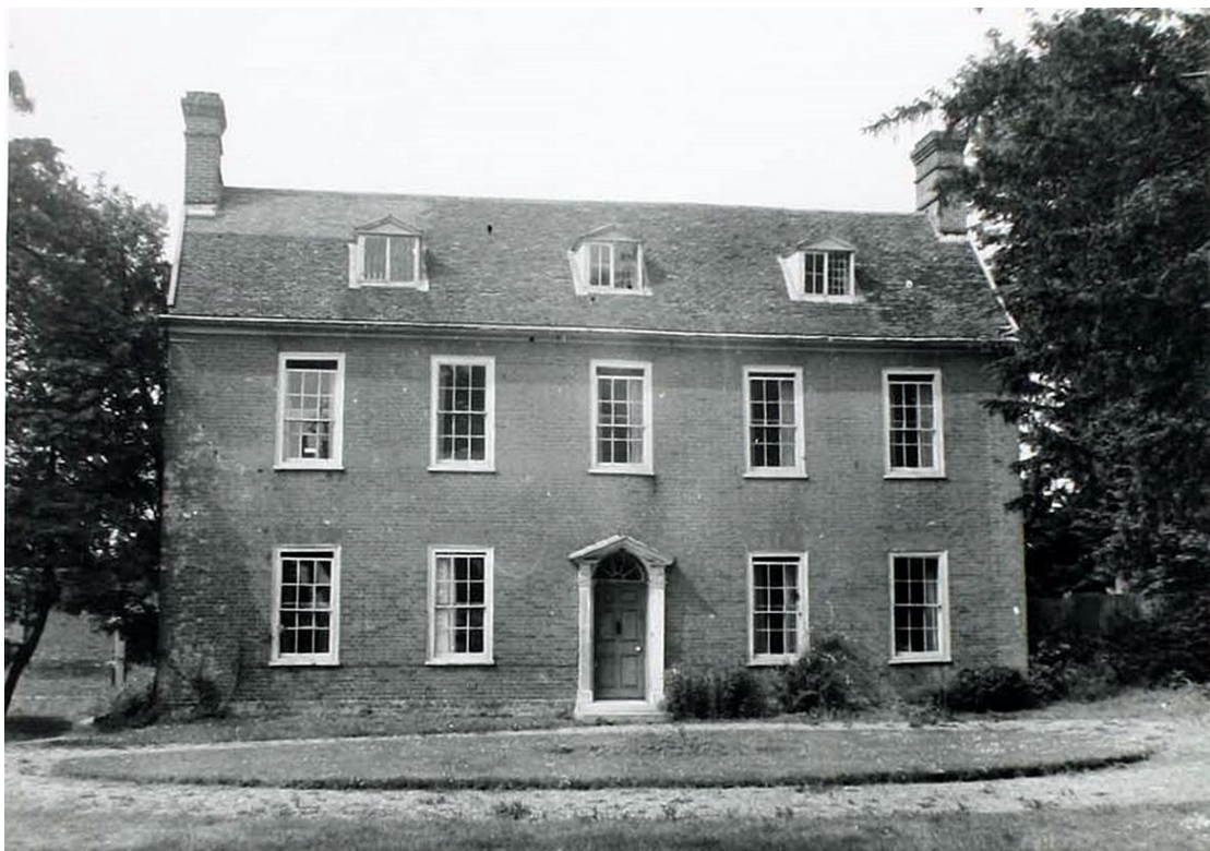
Figure 11. The house in 1949 (Historic England archive). The contrast between the small-paned casement windows of the attic dormers and the sashes below is almost certainly an original feature of the building, although some of the former had been replaced with larger panes at this date. They have since been reinstated.
