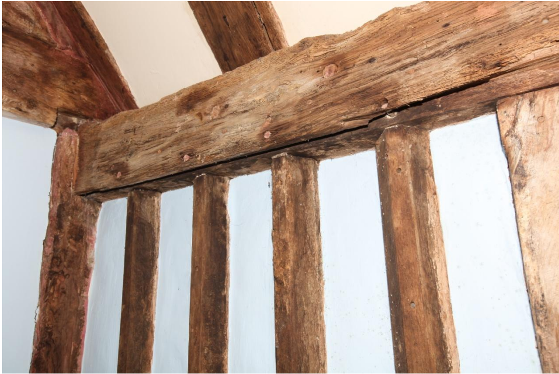
Illus. 21. A detail of the original chamfered window mullions in the back wall of the parlour chamber (illus. 20). Each mullion is tenoned and pegged to the roof-plate, which contains a groove for a horizontally sliding window shutter. Plainly chamfered mullions of this kind are not common and this feature represents a rare survive. Illus. 15 shows its weathered sill that would have projected through the original external render.
