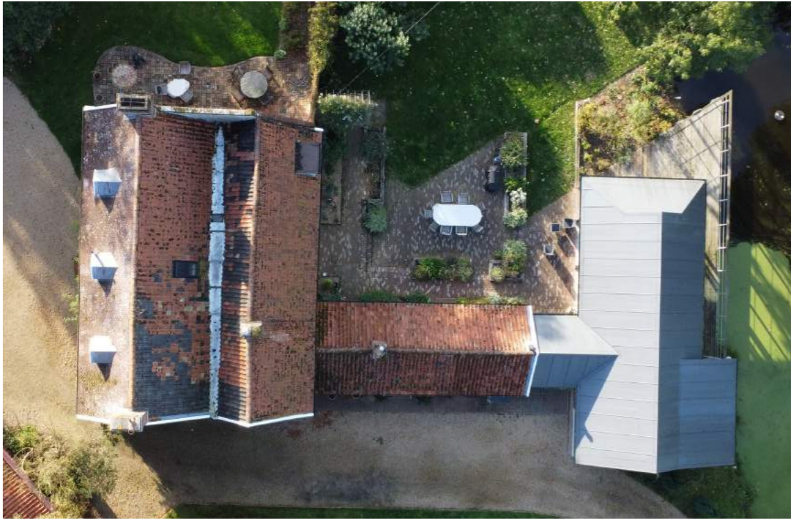
Drone shot from birds eye view showing the site against the existing survey plan
