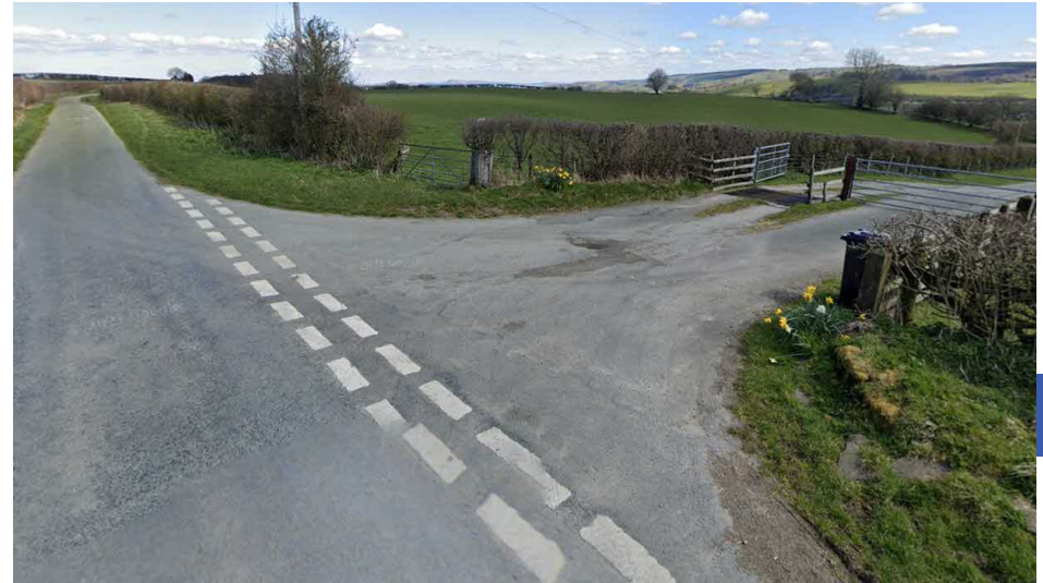
Existing Access and Visibility
