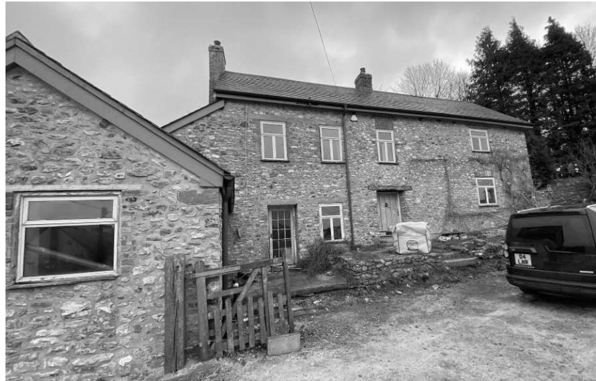
Fig 2: Higher Seavington Farm viewing North.
