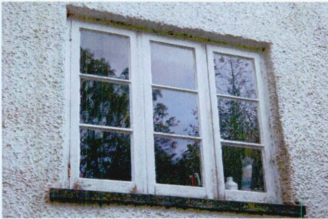
Left: 1920's window to family bathroom
