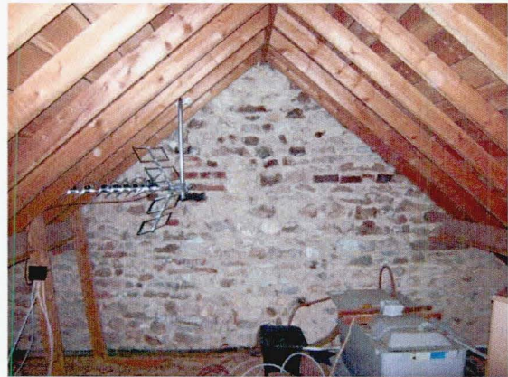
Above: Roofspace over main bedroom and bathroom, showing former external gable (?) and roof scar at low level, against brick-nogged king post truss
