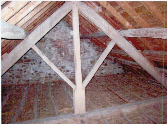
Above: the eastern roofspace, showing the C18/early C19 trusses and purlins. Note brickwork to far gable, evidence of a lost chimney and fireplace
