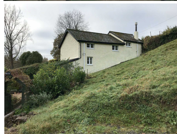
View of house from East
