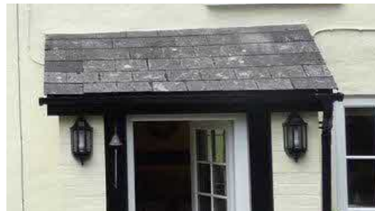
EXISTING PORCH ROOF
