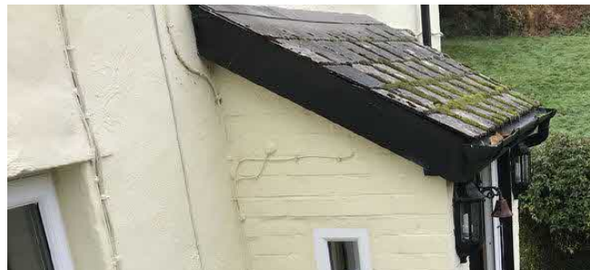
EXISTING PORCH BARGE BOARD
