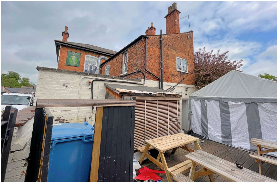
PHOTOGRAPH LOOKING NORTH TO REAR OF PUB FROM EXTERNAL TRADE AREA
