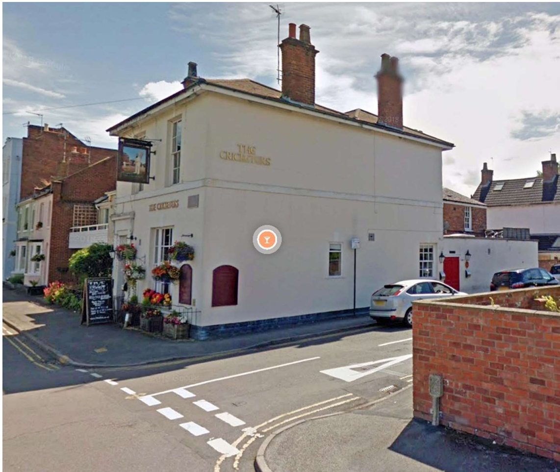
PHOTOGRAPH LOOKING SOUTH WEST FROM ARCHERY ROAD TO SIDE ELEVATION
