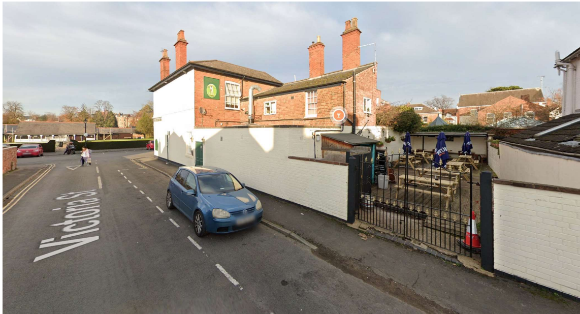
PHOTOGRAPH LOOKING NORTH EAST TO REAR OF PUB, ARCHERY ROAD BEYOND
