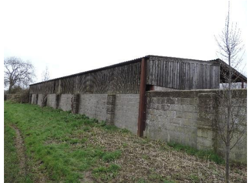
Plate 5: Shed 2 Viewed from Northeast
