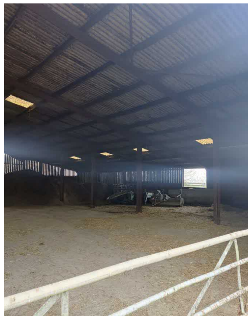
Figure 5 - Internal view from SE
