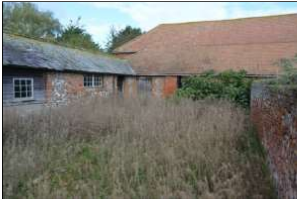
Plate 111: West Range from the southeast
