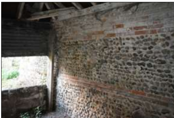
Plate 130: CS4: view to southwest
