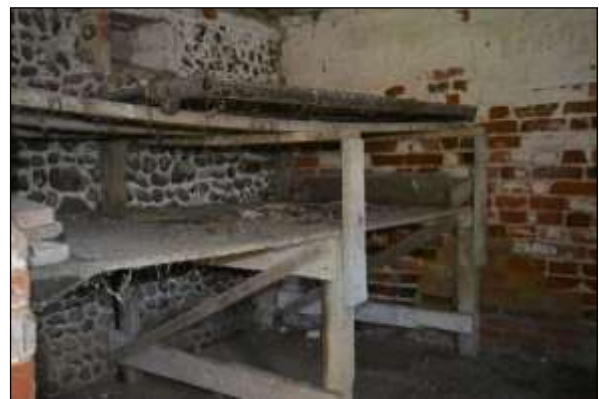
Plate 108: E3: view to southwest
