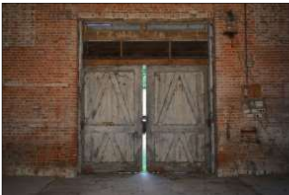
Plate 90: Double doors in north wall
