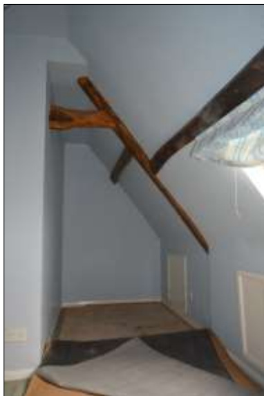
Plate 54: Room S2: view to west
