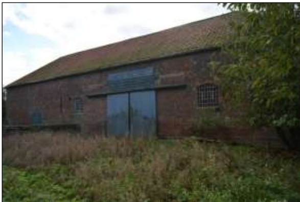
Plate 82: Barn: north elevation
