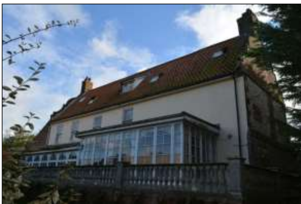
Plate 3: North elevation from the northwest
