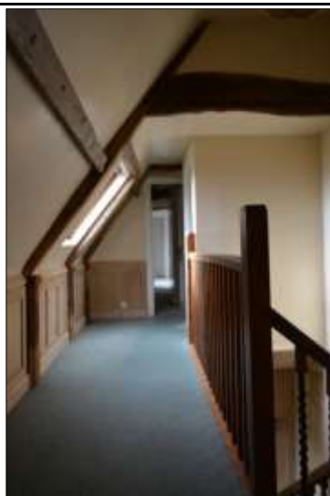
Plate 57: Room S4: view to west
