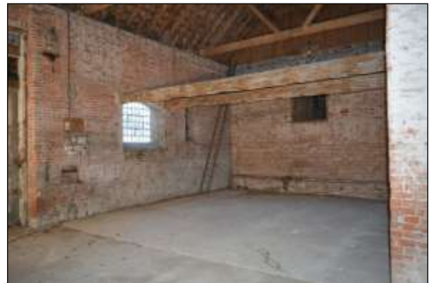
Plate 89: Barn interior: northeast corner
