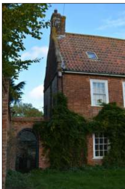
Plate 8: West elevation from the southwest
