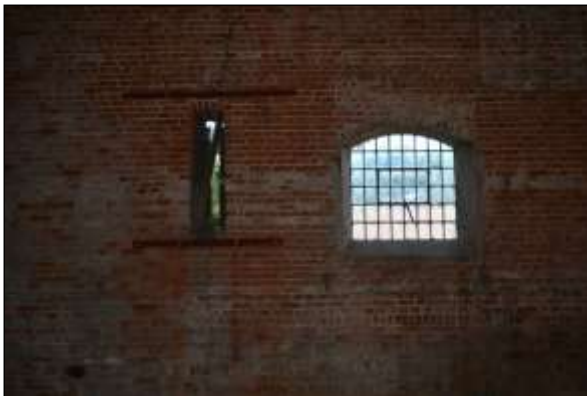
Plate 94: Barn: window and windeye detail
