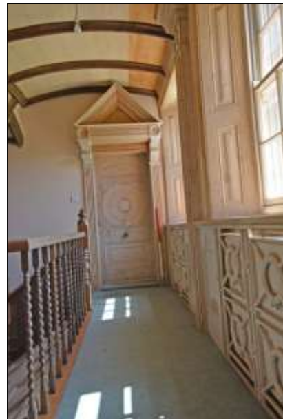
Plate 33: F1: view to east
