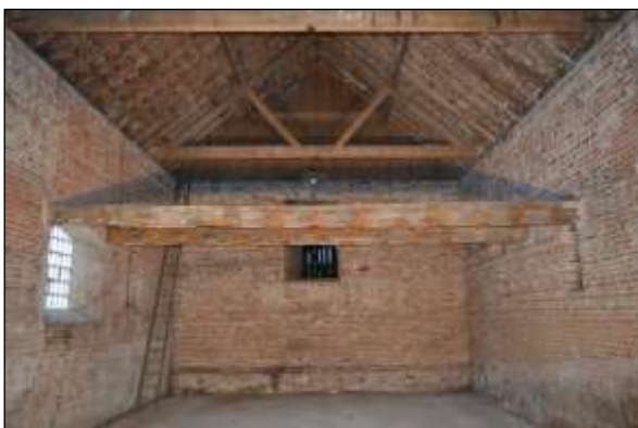
Plate 86: Barn interior: view to east
