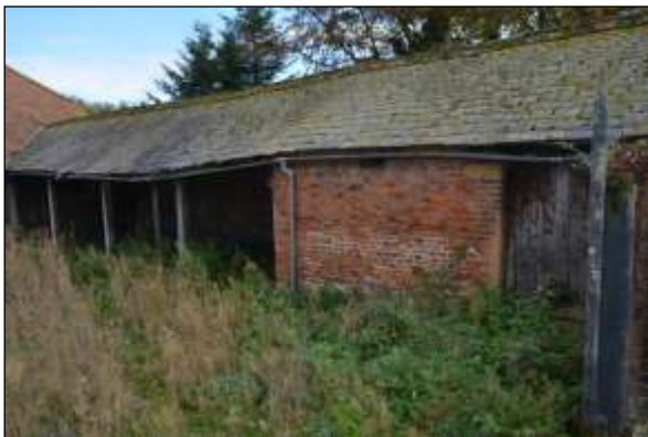
Plate 101: East Range: view to north east
