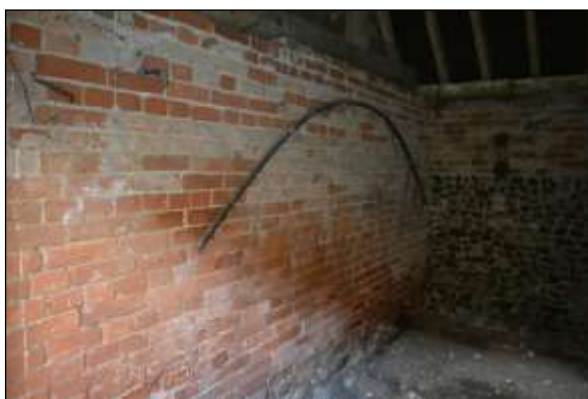
Plate 124: CS2: west wall
