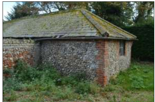
Plate 102: East Range: southern extent
