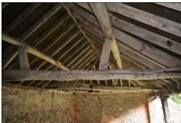
Plate 122: CS1: roof truss
