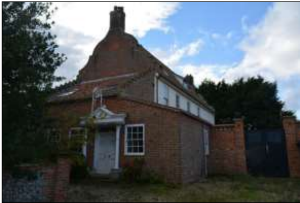
Plate 6: East elevation from the northeast
