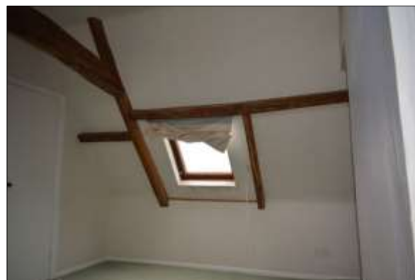
Plate 68: Room S8: south wall
