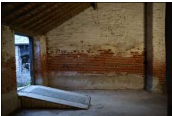
Plate 96: B2: view to west showing ramped entrance
