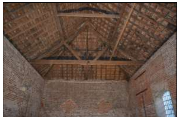
Plate 93: Barn: roof Truss
