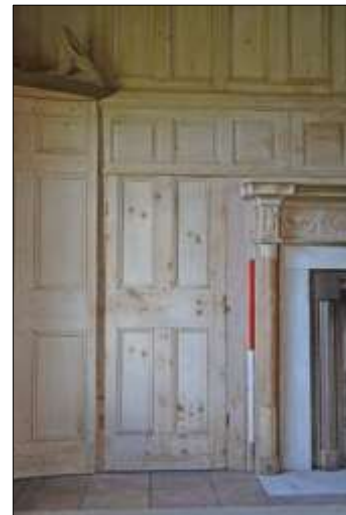
Plate 17: G1: re-used door as panelling in west wall
