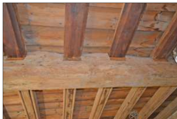
Plate 28: G5: joists detail
