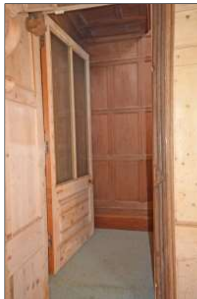
Plate 21: G2: door to stairs and panelling beyond
