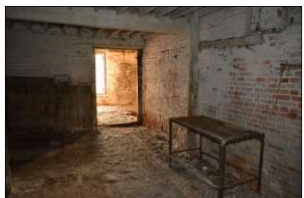
Plate 99: B3: view to south
