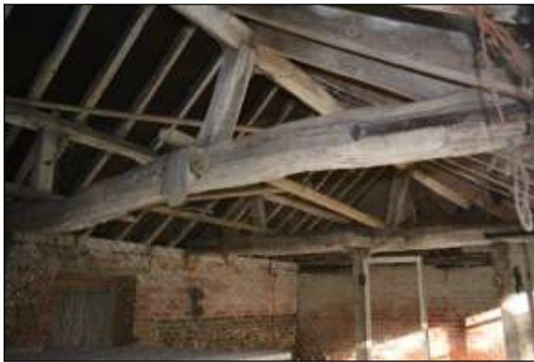
Plate 128: CS3: roof truss
