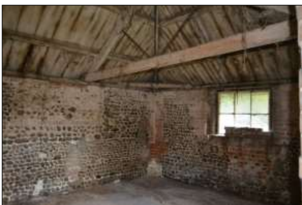
Plate 109: E4: view to southwest
