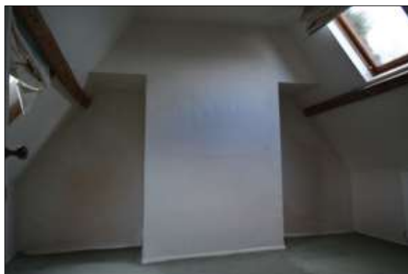
Plate 67: Room S8: west wall
