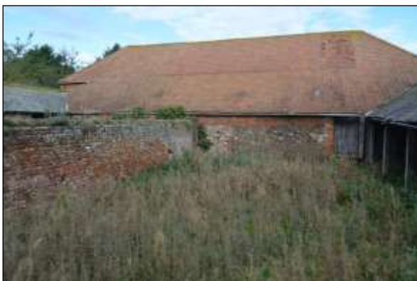
Plate 80: Barn: south elevation, east end
