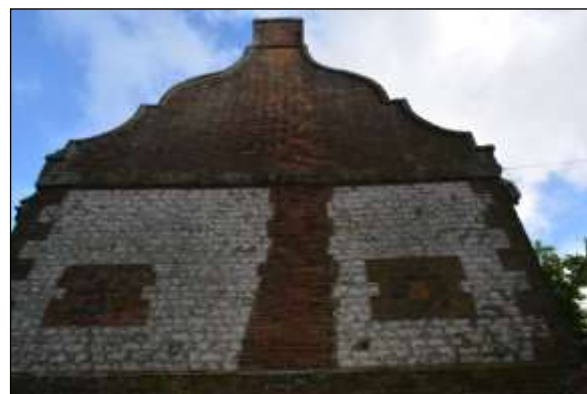
Plate 10: West elevation: Upper section
