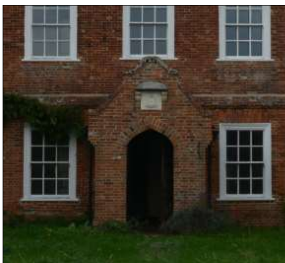
Plate 2: South elevation: porch detail
