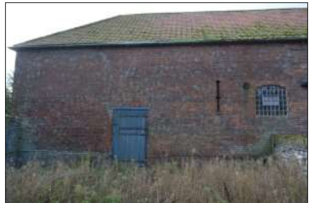
Plate 83: Barn: north elevation, east end
