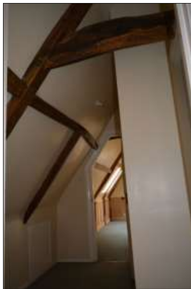
Plate 56: Room S3: view to west
