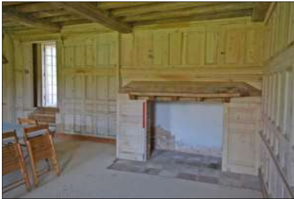
Plate 14: G1: north wall & fireplace
