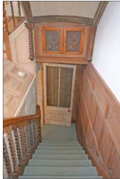
Plate 35: F1: view down the stairs
