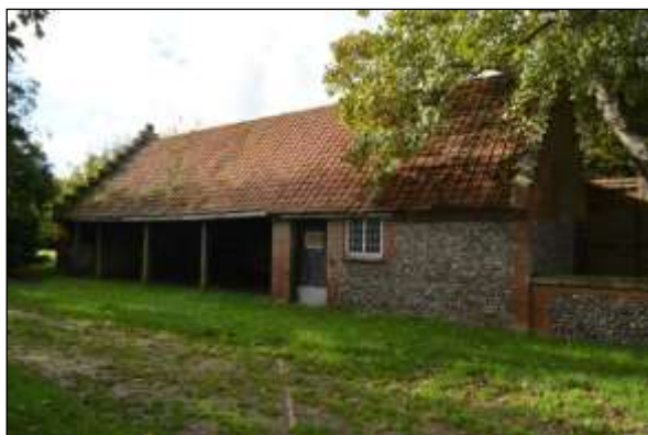
Plate 72: Cart shed: east elevation from the northeast
