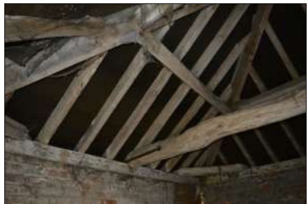
Plate 131: CS4: roof detail
