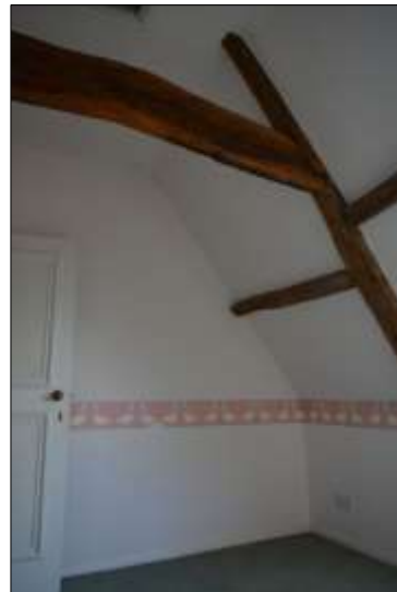
Plate 65: Room S7: northwest corner
