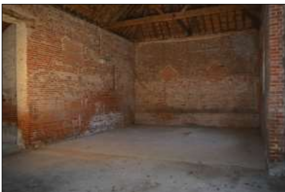
Plate 92: Barn interior: southwest corner
