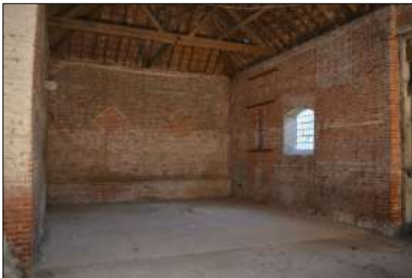
Plate 88: Barn interior: northwest corner
