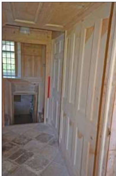
Plate 22: G3: view to north
