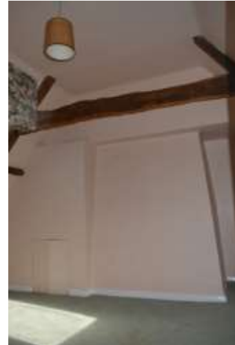
Plate 52: Room S1: east wall
