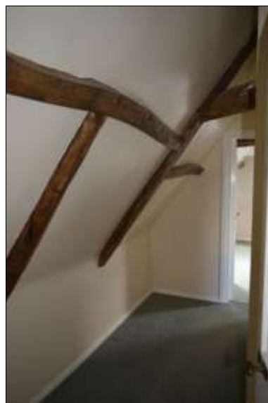
Plate 63: Room S6: view to west
