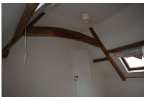
Plate 69: Room S8: southeast corner
