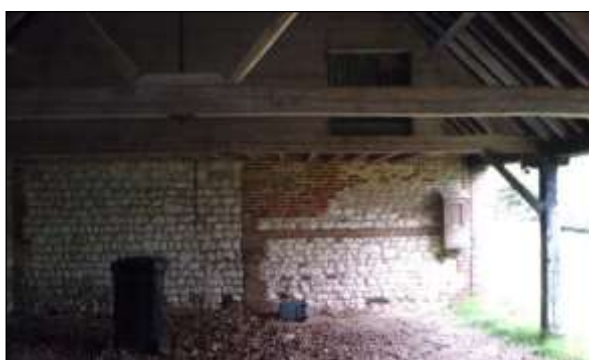
Plate 74: Cart shed: C1: north wall
