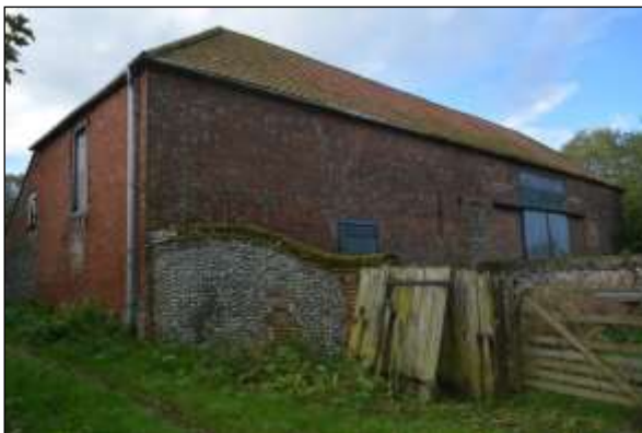
Plate 84: Barn from the northeast
