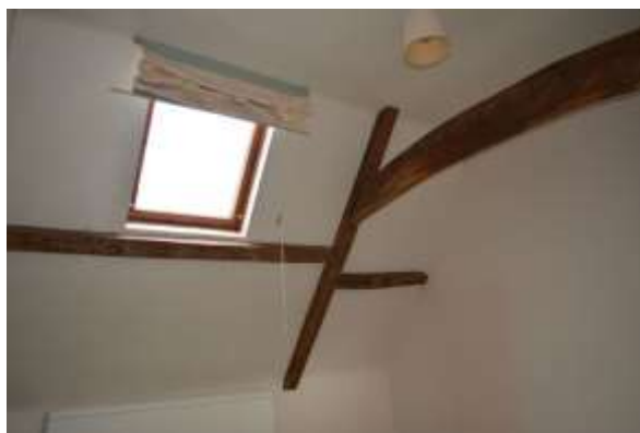
Plate 70: Room S8: southwest corner
