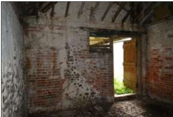
Plate 105: E2: view to southwest
