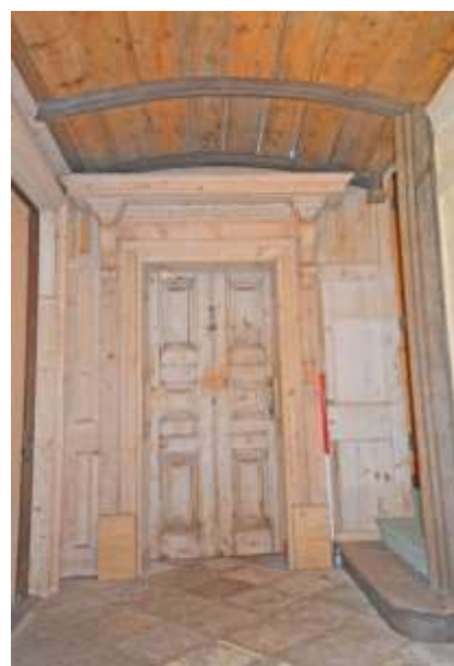
Plate 19: G2: view to west
