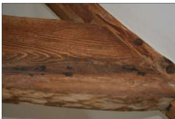
Plate 71: Room S8: carpenter's assembly marks
