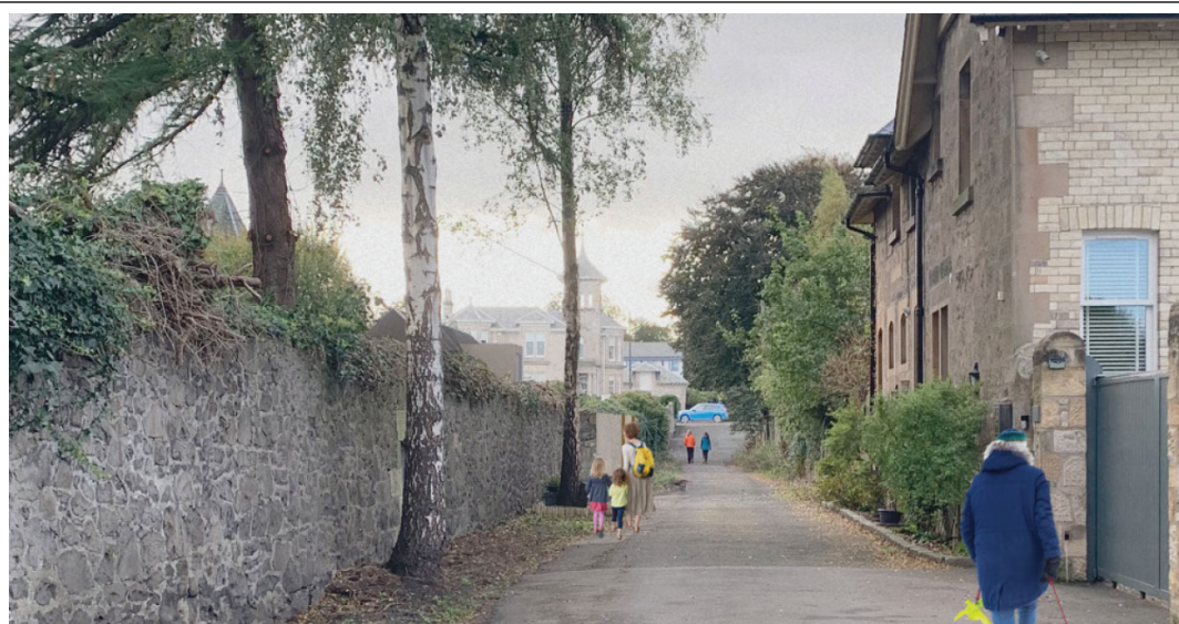
Looking south along Gladstone Place Lane towards Snowdon Place with the proposals in situ on the left-hand side to the rear of 11 Melville Terrace. Gladstone Place Lodge s visible to the right hand side.
