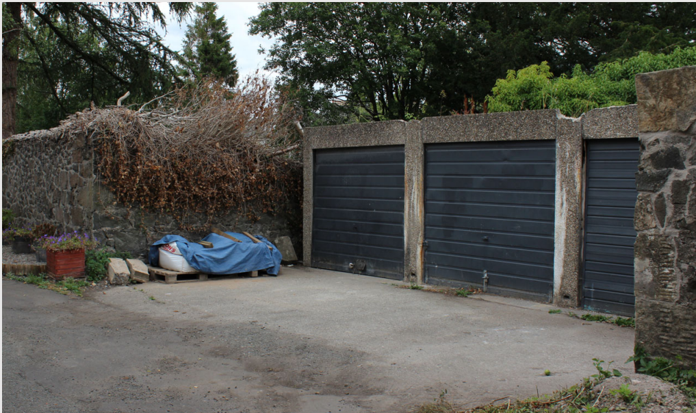
Existing Garage and hardstanding. Much of the rear boundary wall was demolished to create this parking area.
